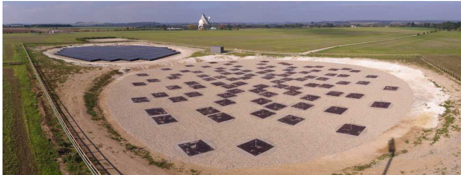
Figure 1.10: The international Low-Frequency Array (LOFAR) station in the UK. The Low Band Antennas, a ‘droopy-dipole’ design, can be seen in the foreground. The High Band Antennas are under the black weatherproof covering in the background. (Image from astron.nl ).
