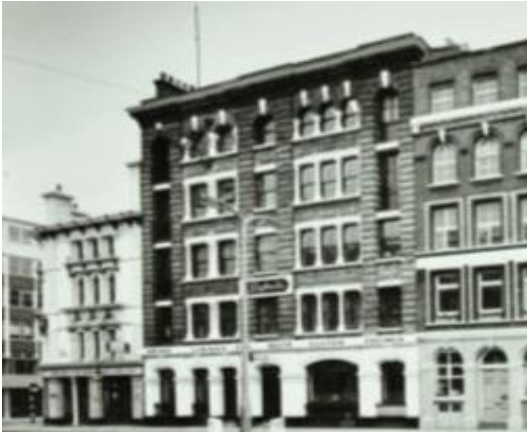
Plate 253. 56-58 Southwark Street (before alteration), Tillot and Chamberlain, architects. Image: LMA
