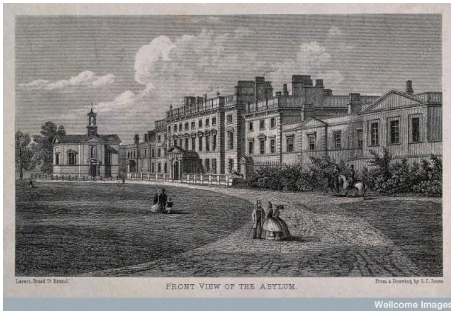
Plate 230. Brislington House Asylum as re-fronted and extended in 1851. Image: Wellcome
