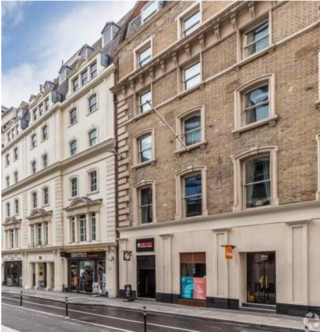
Plate 193. Buildings on Cannon Street (1846-1854) J. Bunstone Bunning. Lower three storeys of each by Bunning (later extended upwards above the cornices). Image: Colliers International
