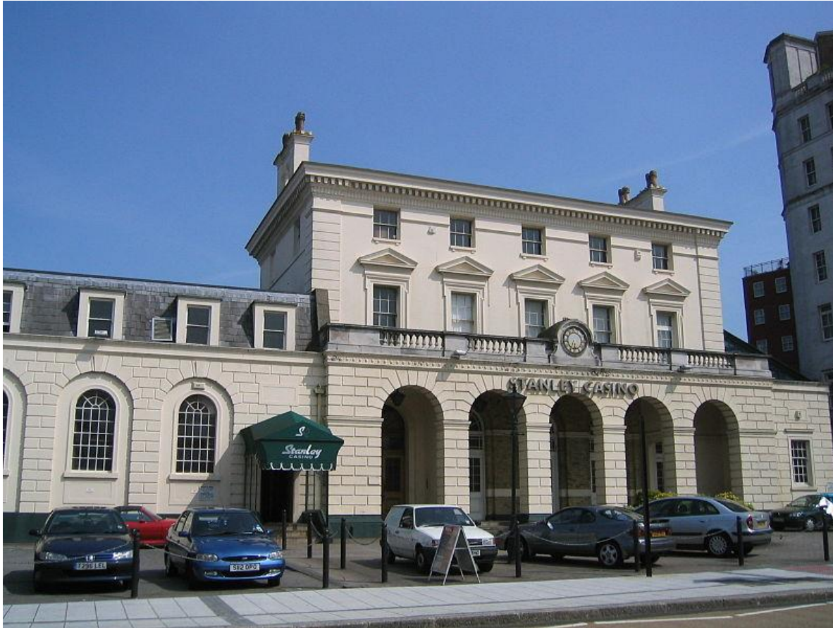
Plate 242. Former Southampton Terminus, Sir William Tite, 1839 (note similarities with elevation of Somerset House seen in Plate 52). Image: Wikimedia Commons
