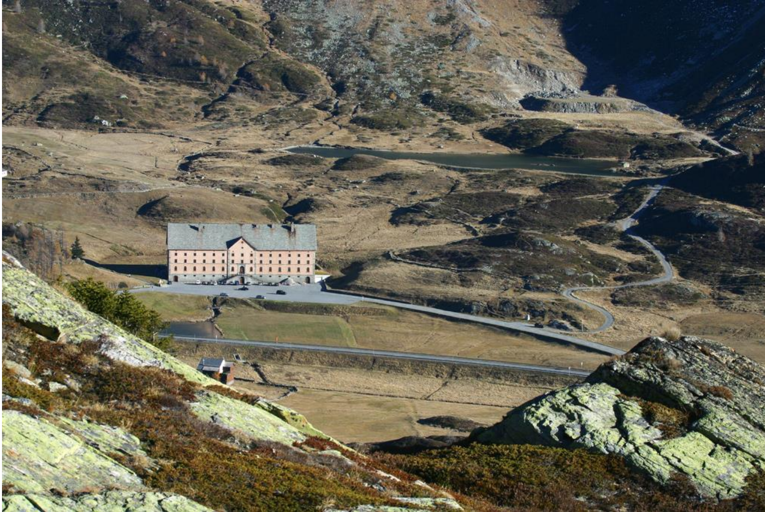
Plate 49: Simplon Pass at the Simplon Hospice, Valais, Switzerland, road and hospice built in 1801, works overseen by Nicolas Céard. Image: Wikimedia Commons
