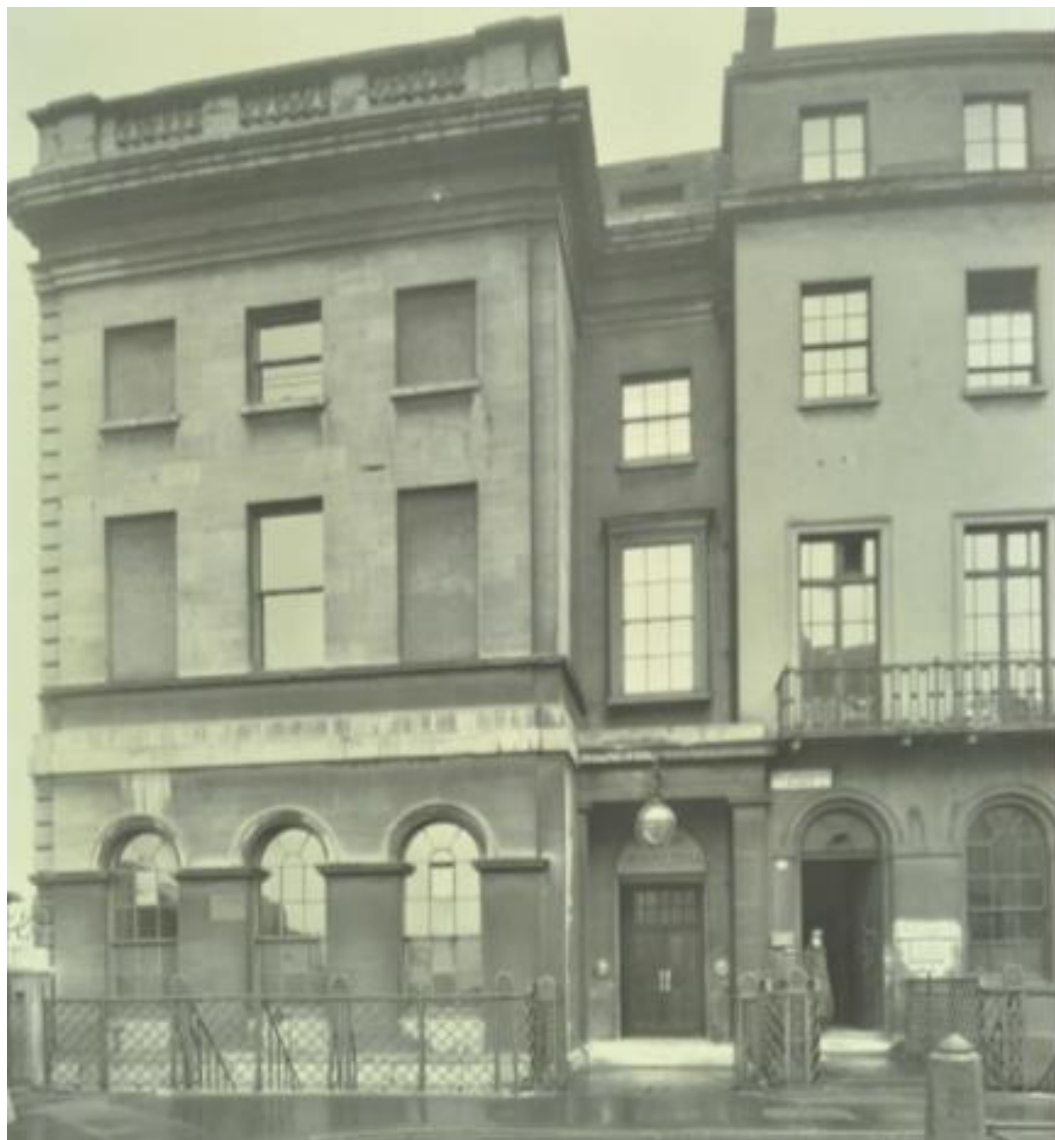
Plate 178. Lancaster Place offices, end bay Robert Smirke, 1817-182. Image: LMA
