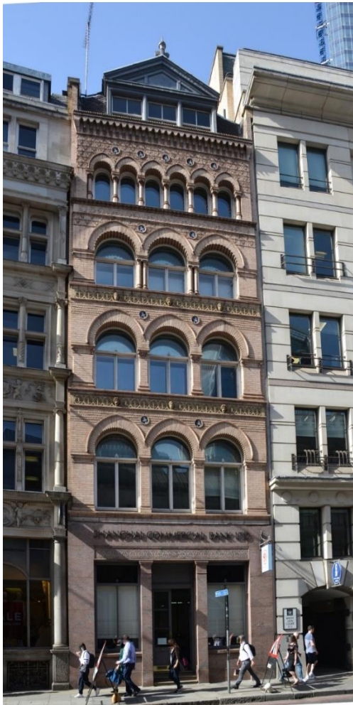
Plate 222. 65 Cornhill London, Edward I'Anson, Terracotta and Portland cement, 1868-1870. Image: Wikimedia Commons
