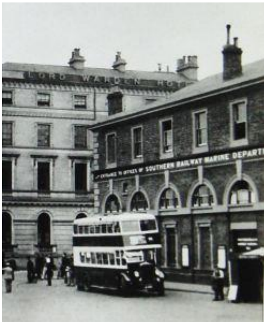
Plate 134. Dover Station, 1844 (and Lord Warden Hotel, 1850). Image: disusedstations.org
