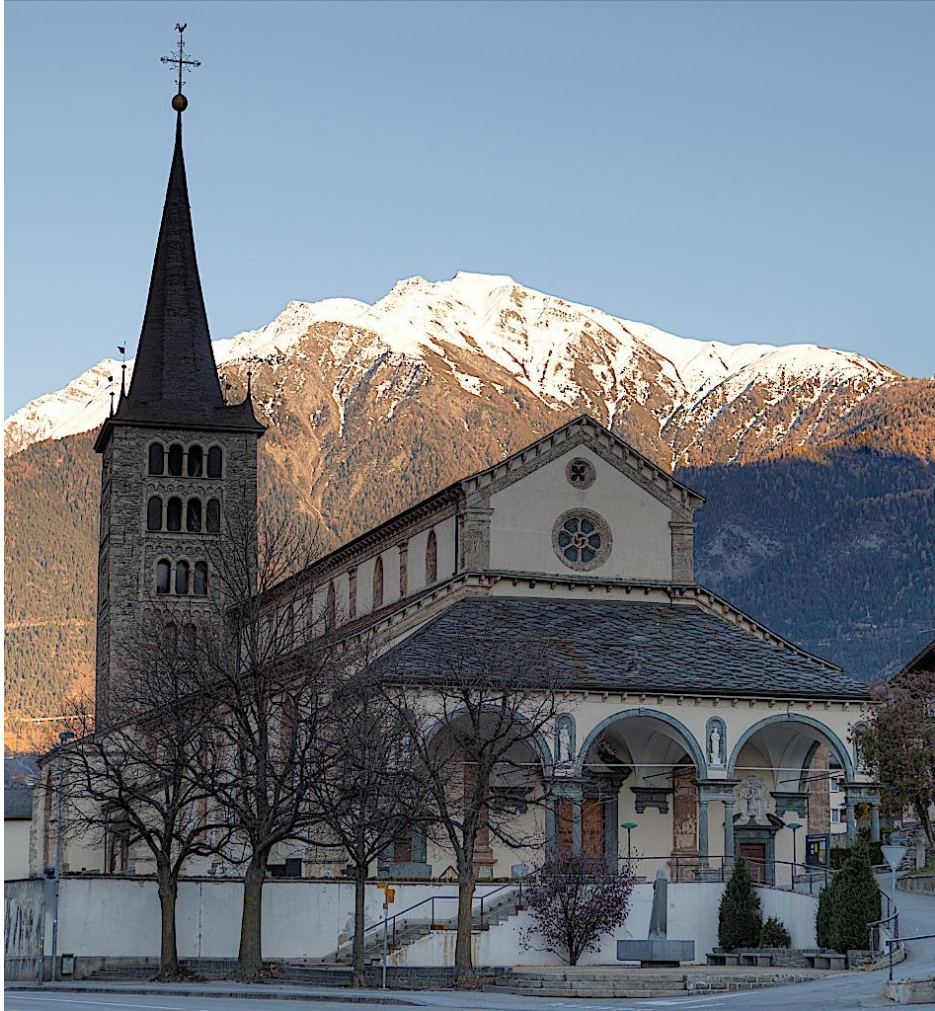
Plate 34: Church of Mariä Himmelfahrt in Glis, municipality of Brig-Glis, Valais, Switzerland, remodelled 1648 to 1668 by the Bodmer brothers. Image: Wikimedia Commons
