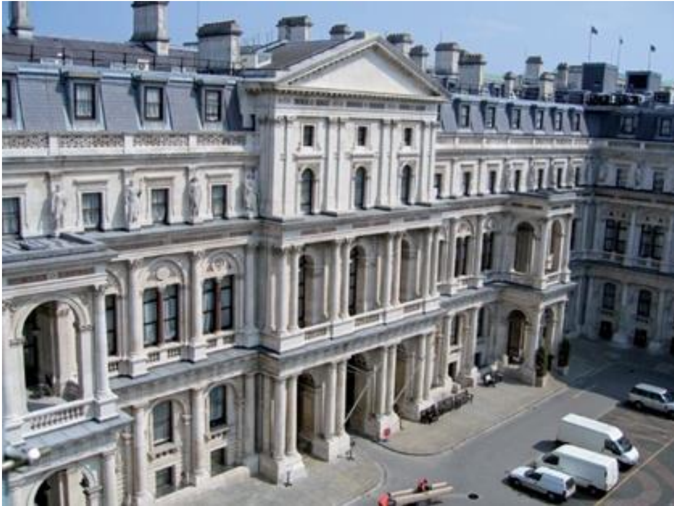
Plate 260. Main Quadrangle to the Foreign Office, Gilbert Scott (designed and built 1861-1870). Image: Geograph.org
