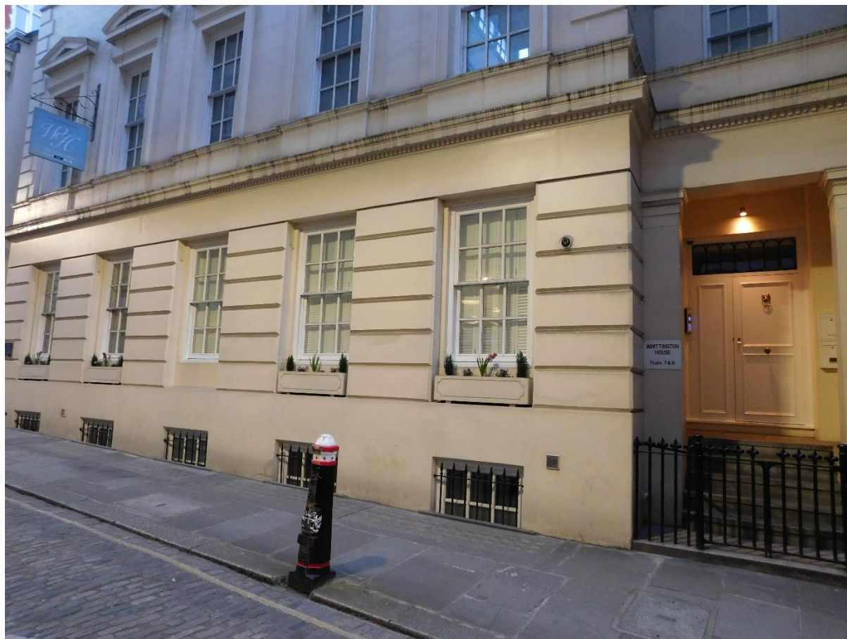
Plate 31: Former Mercer's School, College Hill, City of London. George Smith, c.1830 ground floor detail. Image: author's own
