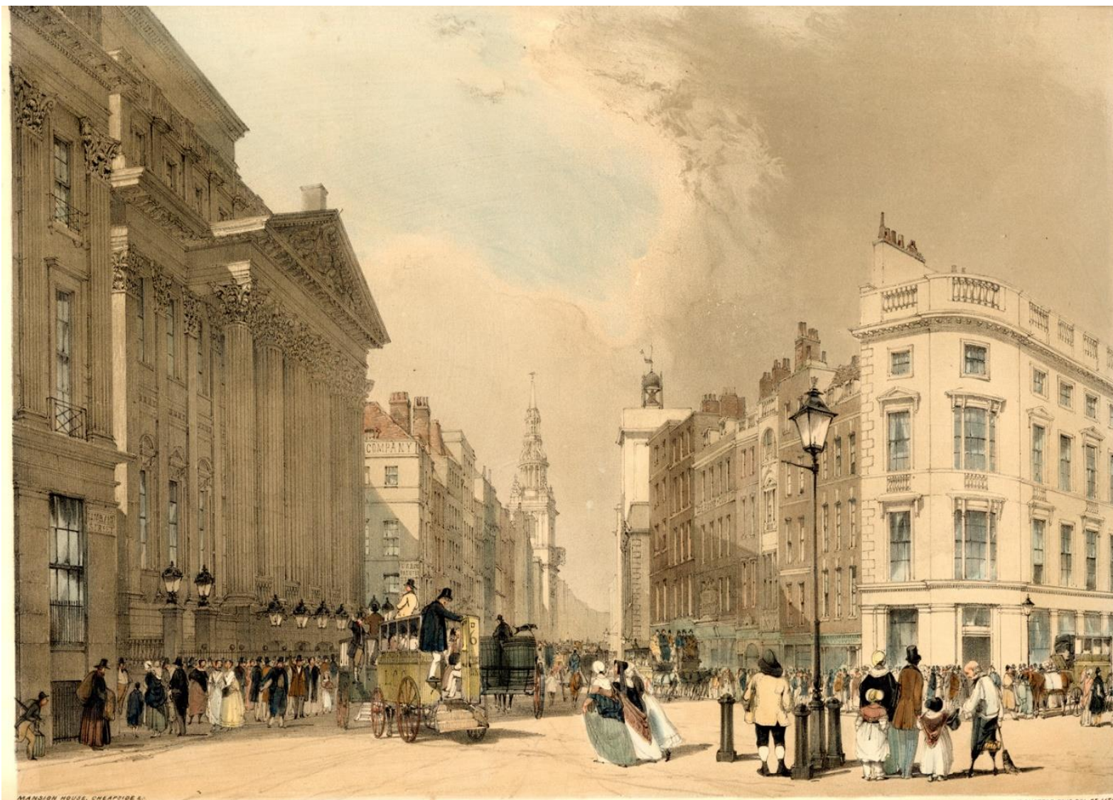
Plate 183. Thomas Shotter Boys, Mansion House, Cheapside, 1842 (Smirke's corner building on the right). Image: LMA
