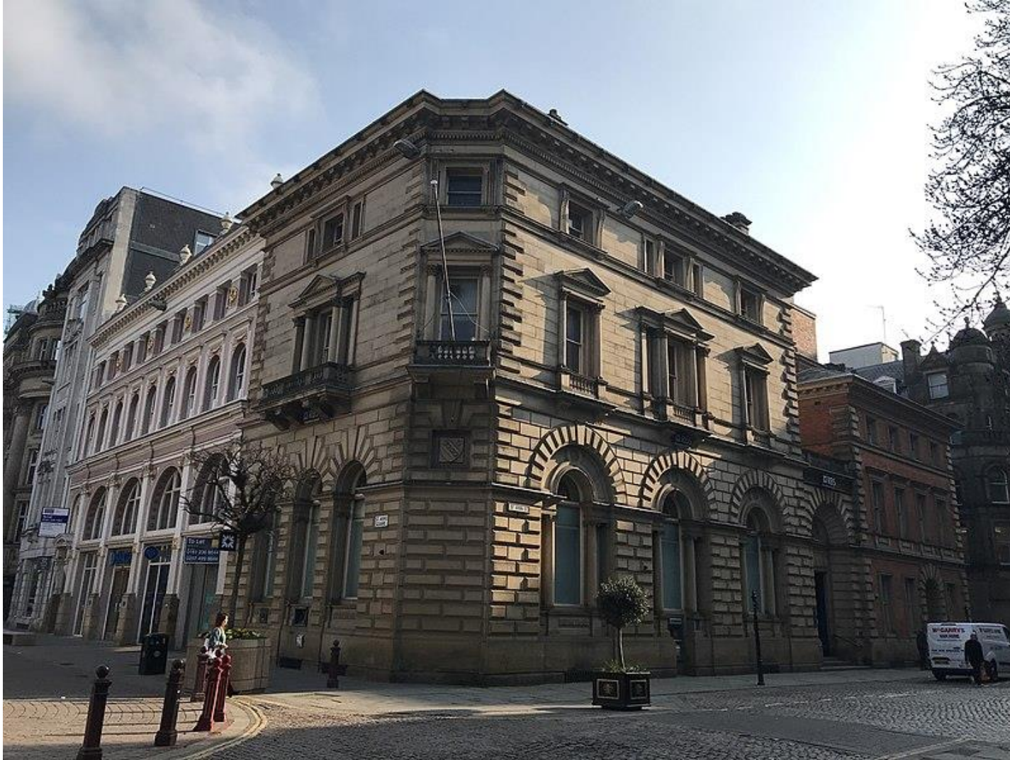
Plate 156. Heywood's Bank and house (to right), St. Ann's Square, Manchester, John Gregan, 1848-49. Image: Wikimedia Commons
