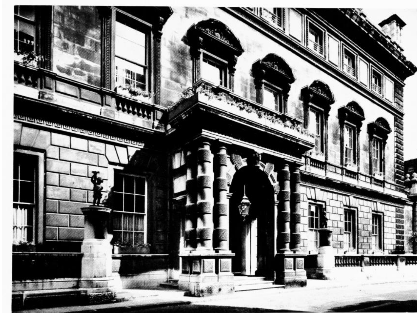
Plate 102. Porch to Bridgewater House, London, Charles Barry, 1840. Image: Survey of London
