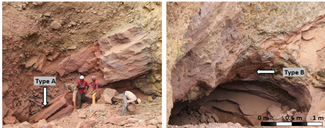
Rock outcrop from which samples Type A and Type B were extracted. Yohannes Amba quarry located near the church complex in Lalibela.
