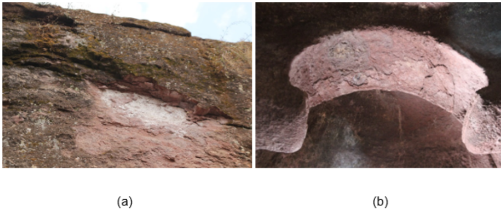
Figure 8.3: Contour scaling on (a) a trench wall Bete Aba Libnos and (b) in the interior Bete Gabriel Rufael
