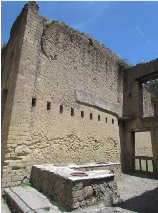
Figure 2.14. Ins. Or. II.6 showing the counter with the four embedded dolia. The beam sockets for the upper floor and some surviving wall plaster are visible on the northern wall. (Author's photograph)
