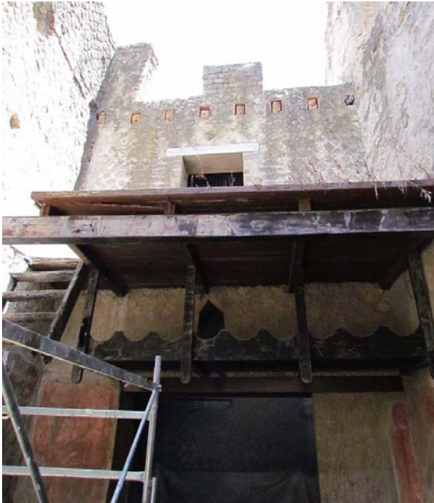
Figure 2.16. Ins. Or. II.9 with the wooden amphora rack and a portion of the staircase still preserved. (Author's photograph)
