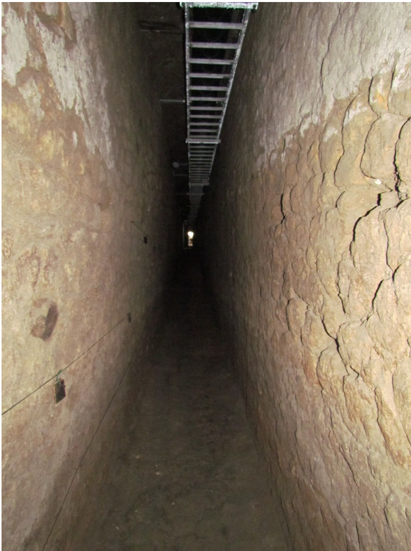
Figure 2.21. Cardo V sewer, looking north towards Ins. Or. II.14 . Note the support for the piping along the ceiling. (Author's photograph)
