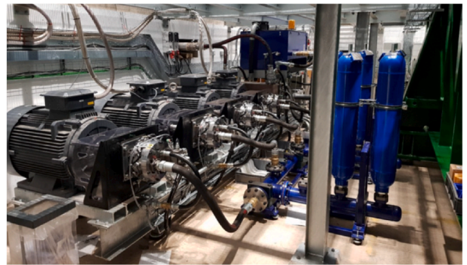
Fig. 5. FastBlade's Digital Displacement hydraulic pumps.
