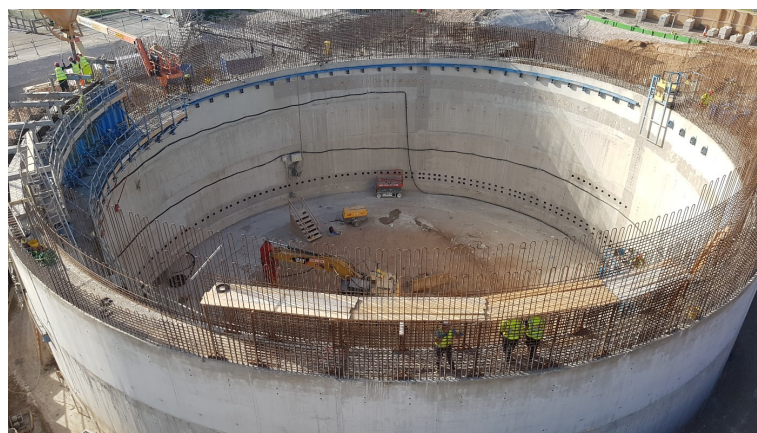
Figure 2.18: Anchorsholme caisson under construction.
