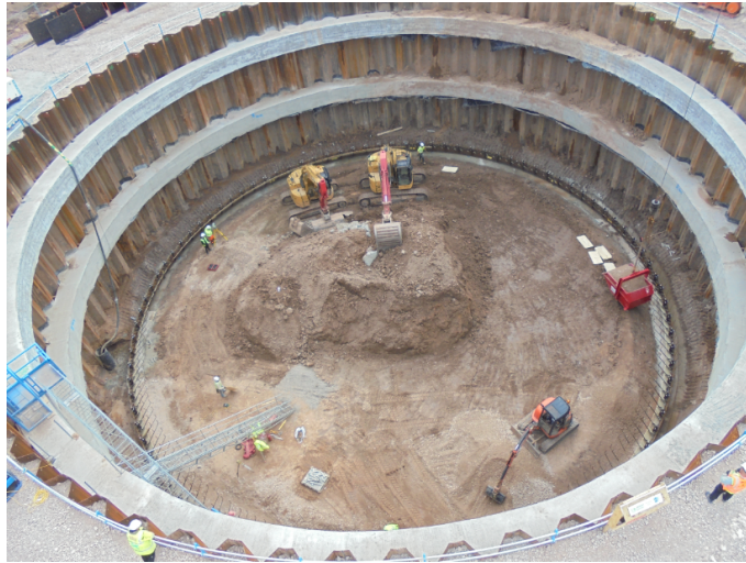
Figure 1.6: Circular sheet pile cofferdam with concrete support beams at Anchorsholme Park.
