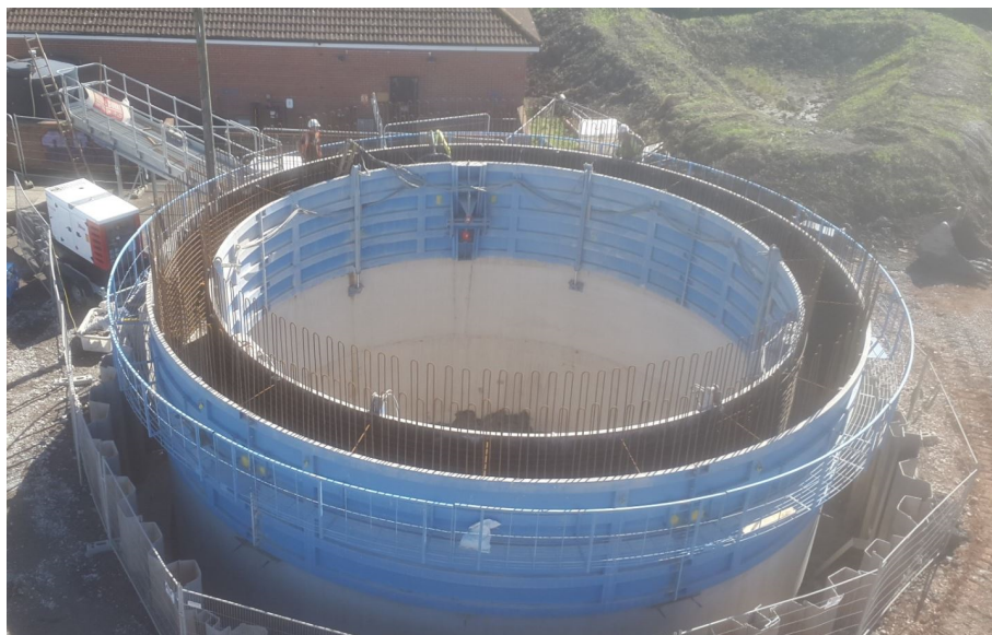
Figure 2.7: Sloway Lane caisson under construction.
