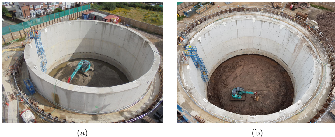
Figure 2.26: Lennox Gate caisson during sinking.
