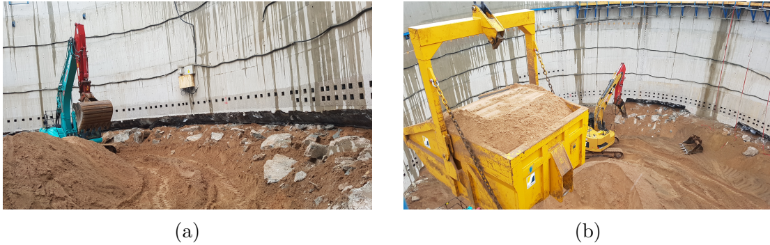
Figure 2.21: Excavation within the Anchorsholme caisson.
