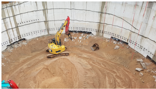
(a) Breaking out Caisson Footing.
