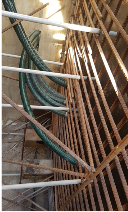
(a) Cable ducts cast in RC wall prior to concrete pour.
