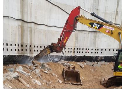
(b) Rock breaker removing footing.
