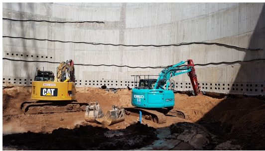
(c) Excavation inside the caisson during sinking.
