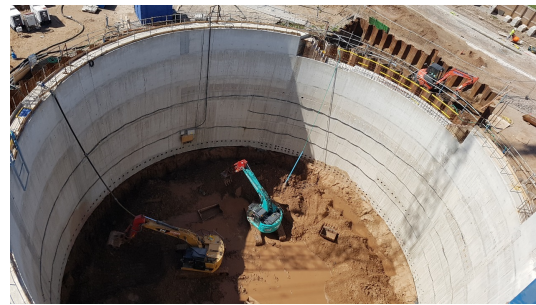
(d) Excavation inside the caisson during sinking.
