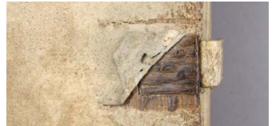
[PLATE 40] Strap anchor to centre of fore-edge of the left board: showing three oak trenails
