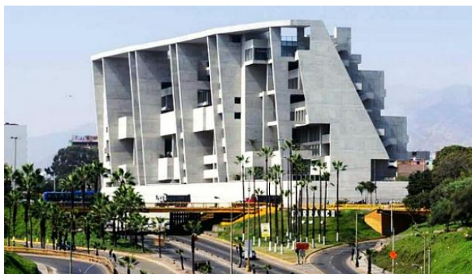
Figure 1. UTEC main building
