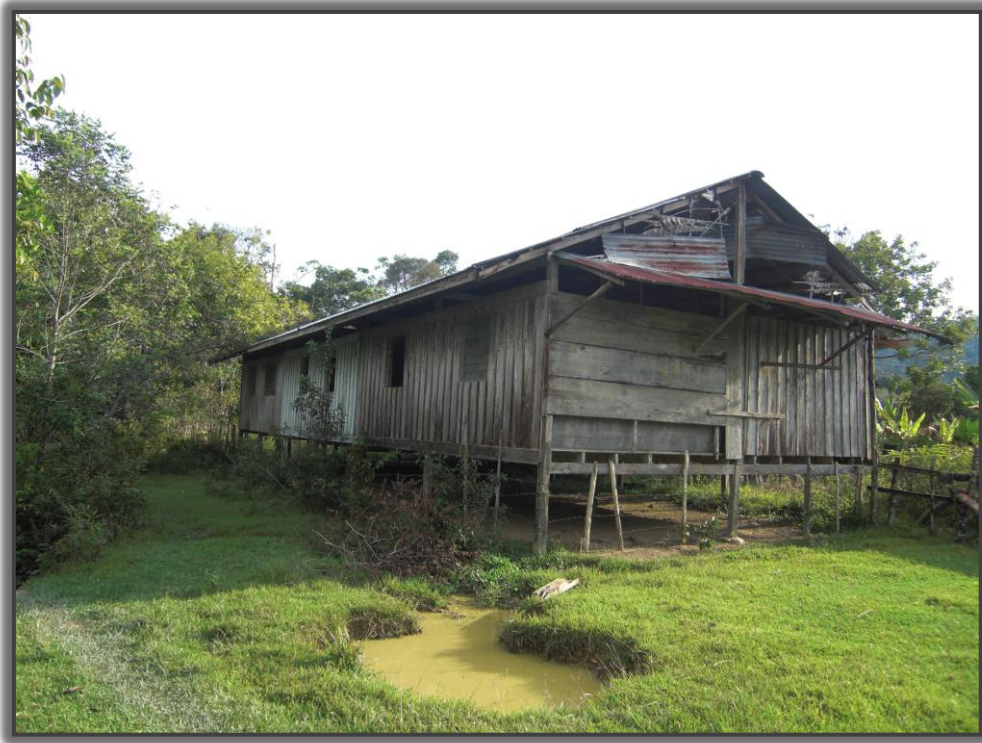
Figure 51: The tawa of the abandoned longhouse at Batu Patong, 2010.
