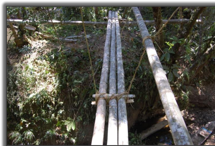
Figure 15: Rattan lashings on the bamboo bridge over the Da'an stream
