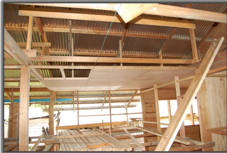
Figure 36: The interior of Judine's new tawa, during the installation of a suspended plywood ceiling to reduce radiant heat from the metal roof
