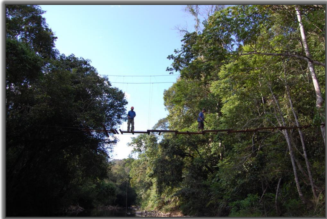
Figure 45: Setting the wires (view from the river)
