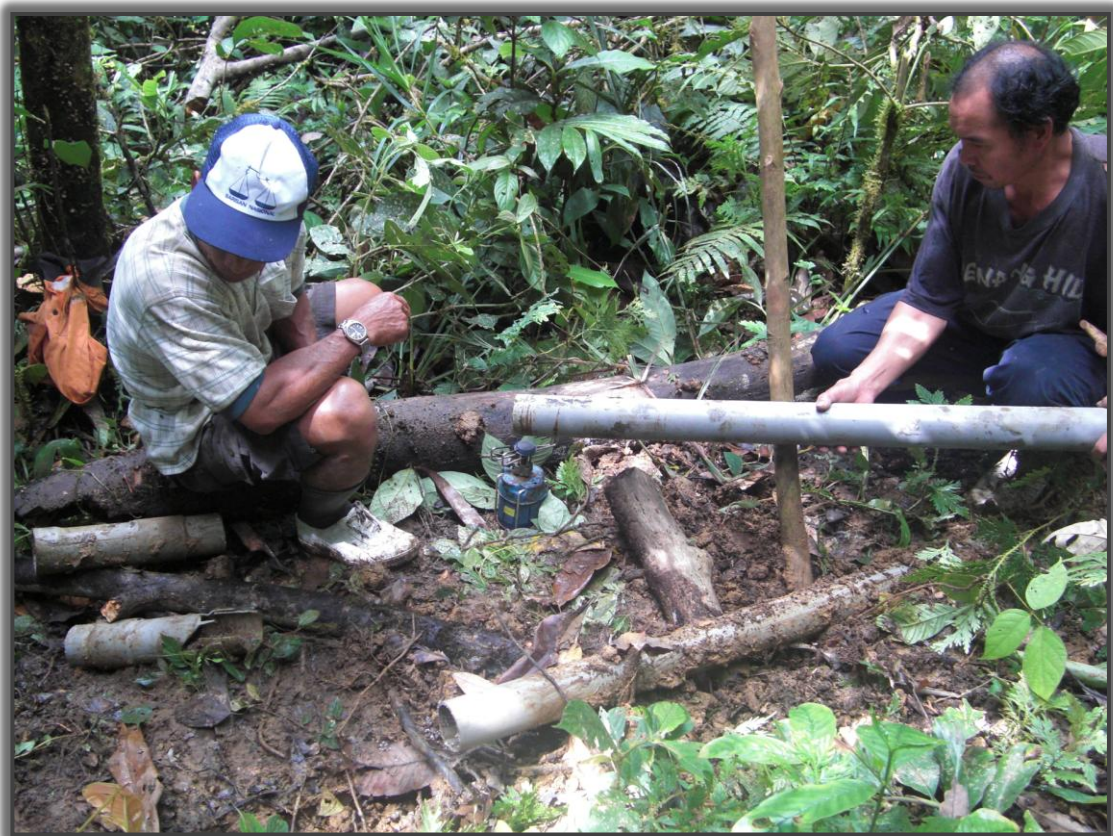
Figure 25: Fixing the waterpipe, done using the forest as a source of tools and materials
