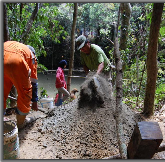
Figure 41: Robert mixing cement
