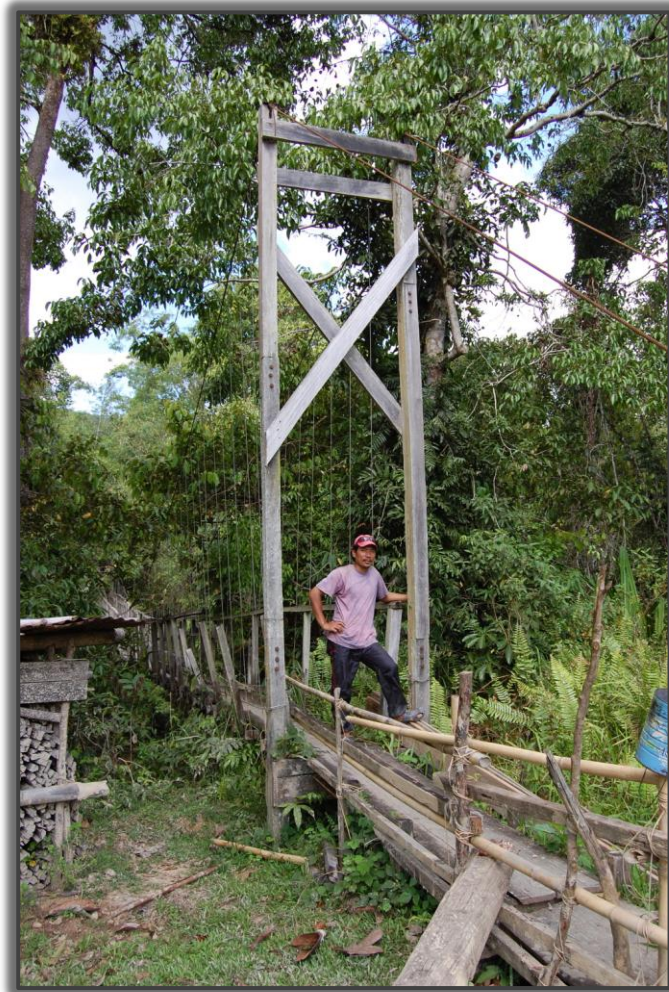
Figure 12: Remudu suspension bridge built by British charity ‘Trekforce’ (compare with the Pa’ Dalih villagers’ bridge in Figures 1 above, and 60 below)
