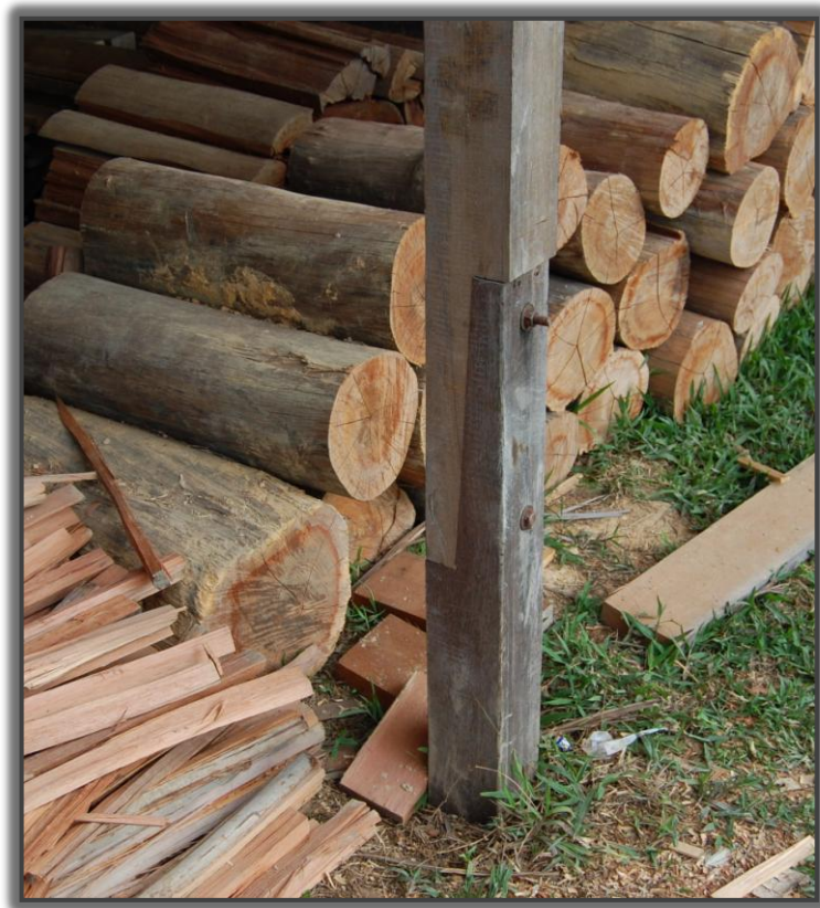
Figure 33: Typical structural support post at the base of the new tawa. The lower part is belian hardwood, and the upper part local wood
