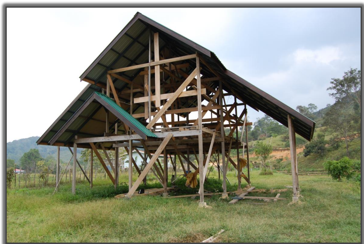
Figure 35: Ganang's new house under construction
