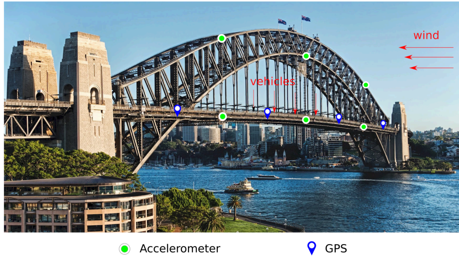
Figure 1.1: Structural Health Monitoring (Sydney Harbour Bridge, modified from source: Arcadis [4])
