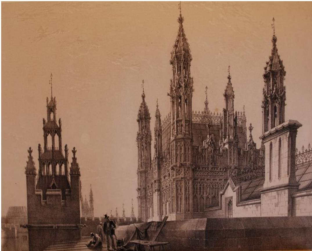
31: Workmen adding the final touches, Ryde, Illustrations , 1849.
