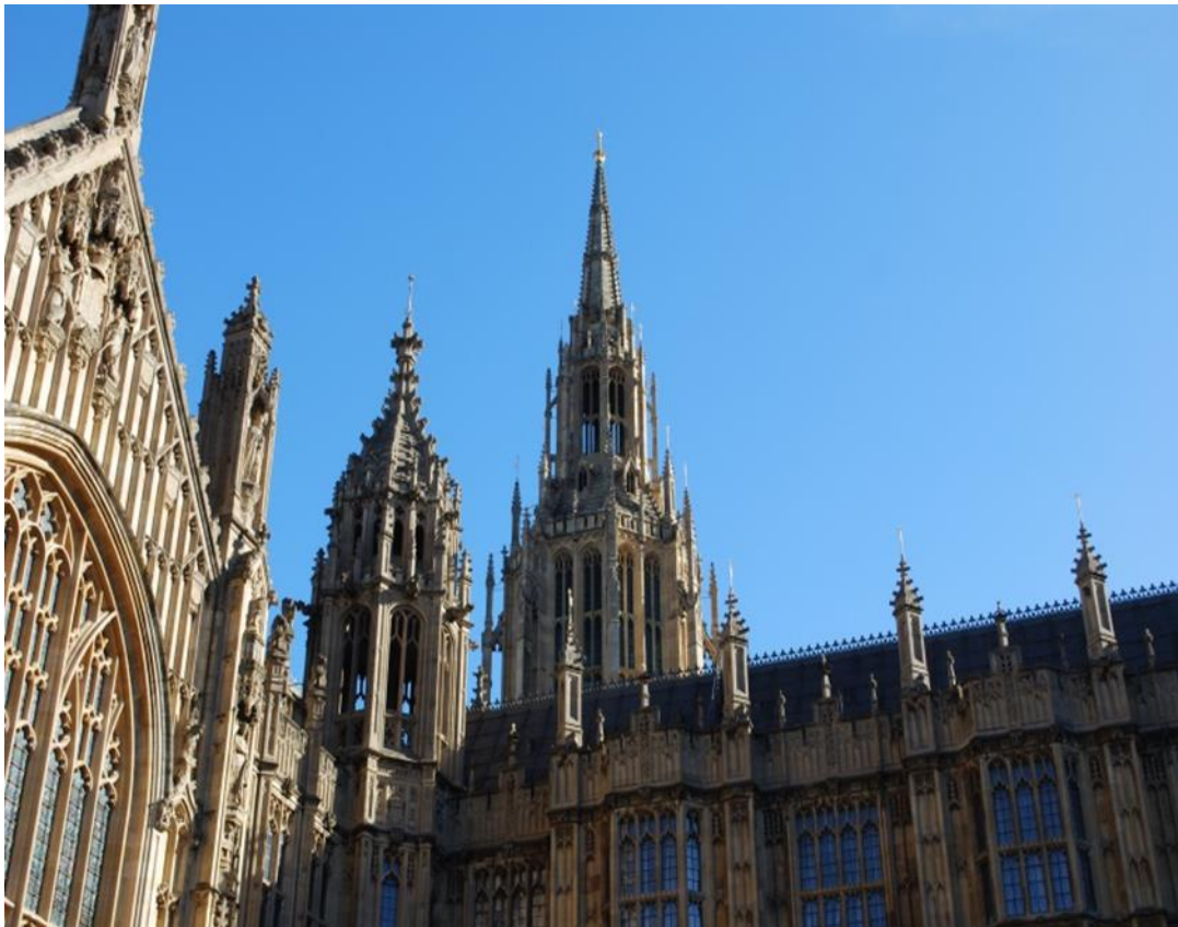
53: The central tower and ventilation shaft, author, 2015.
