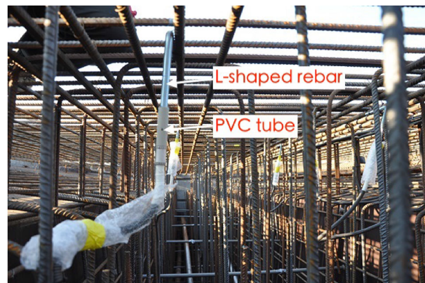
Fig. 5 Mounting SO807 with L-shaped rebar and PVC tube
