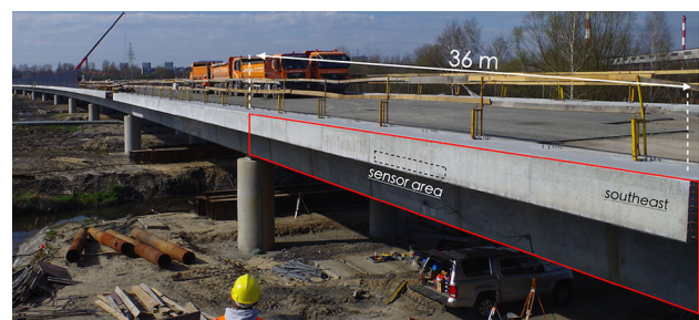
Fig. 3 Monitored bridge span of Gm1-2W at Southeast end
