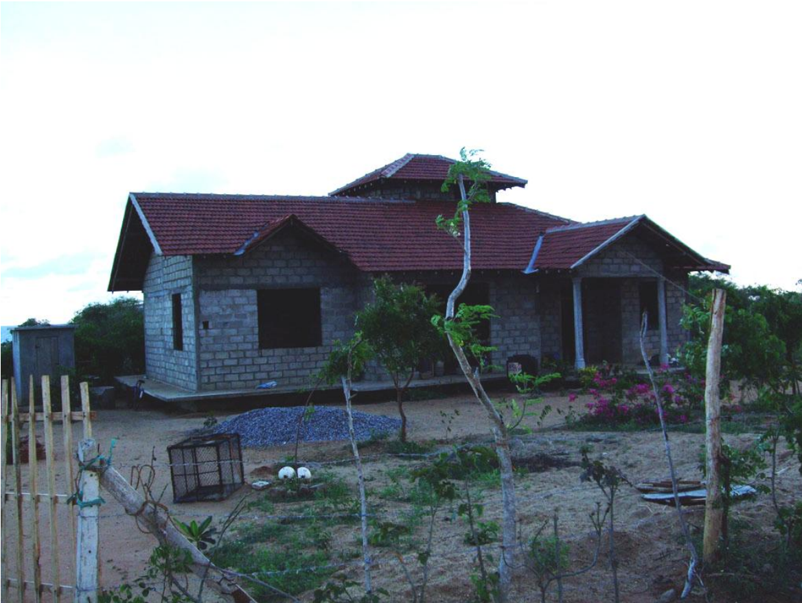
Figure 22. One of 11 houses in the isolated community of Goal Housing, Kirinda.
