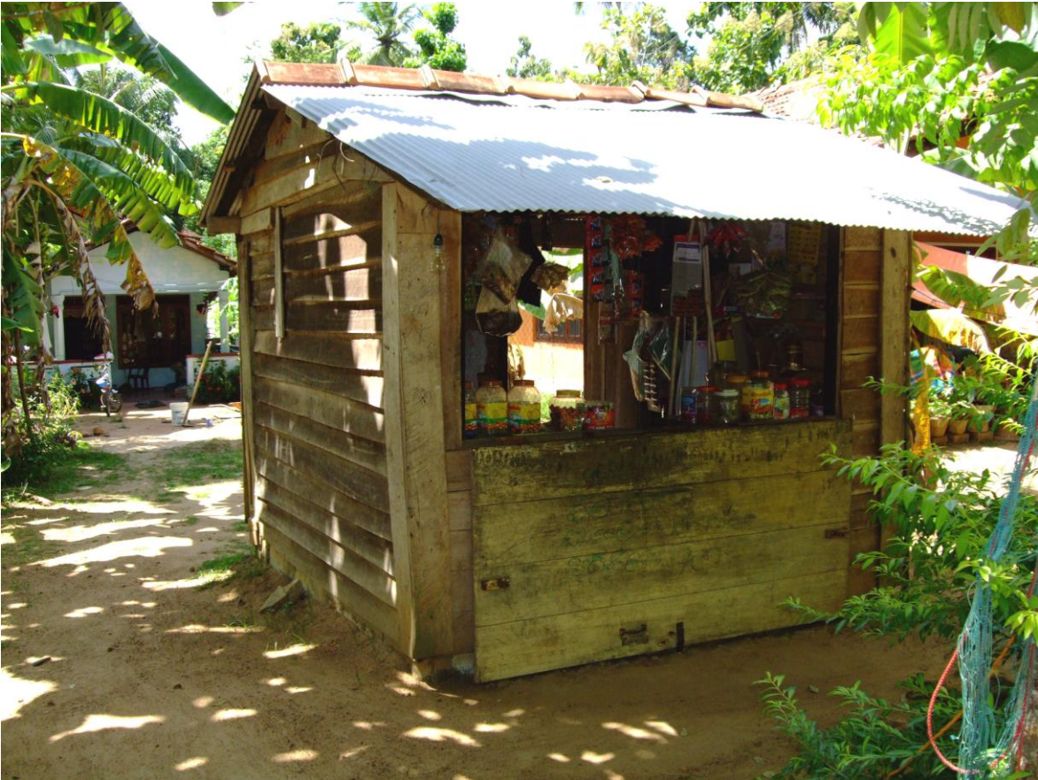
Figure 18. A boutique outside a fisherman's house in Nakulugamuwa Housing, Nakulugamuwa South. It is managed by his wife; an INGO provided her with 20,000 rupees worth of goods to sell, whilst the structure was built through her husband's daily earnings.
