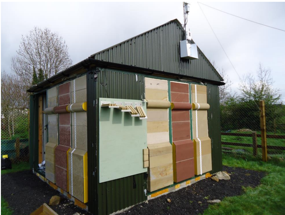
Figure 42: Test structure at Derrygonnelly, Northern Ireland
