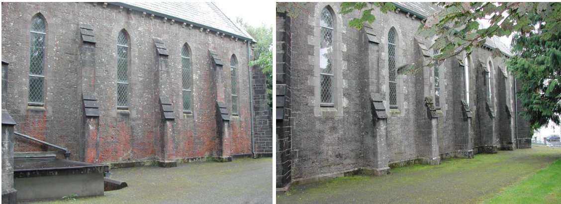
Left) Northern façade, Right) Southern façade. Photos courtesy: Adamson et al. (2009)
