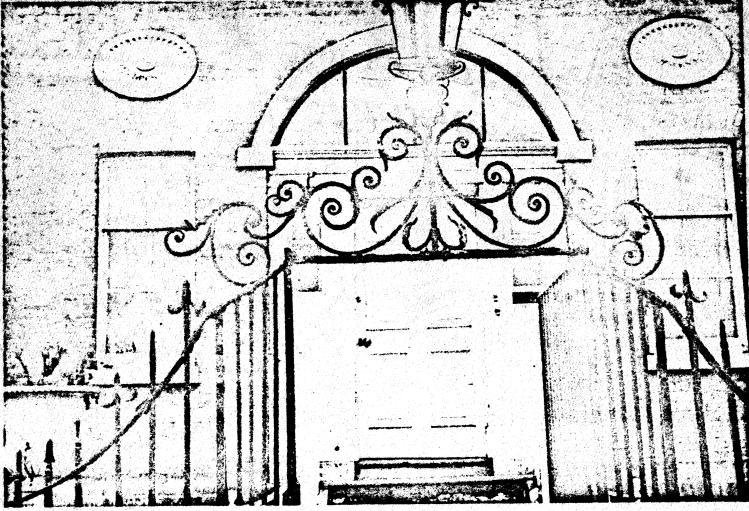
Fig 65 Front door of Kent House, Hammersmith.
