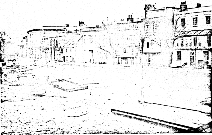
Fig 66 Kent House from Hammersmith Bridge. The house is the bow fronted structure behind the third tree from the right.
