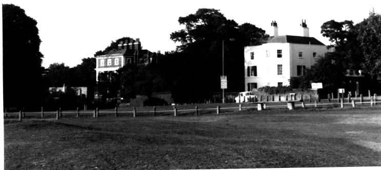
Fig 72 The White House on the right and Park Hall on the left.
