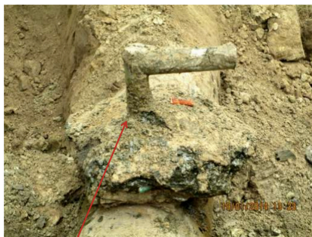
Closeup: Illegal fitting on 28" Nkpoku-Bomu Pipeline right of way at Ekpoko. Picture was taken during Joint Investigation of 19th January 2014.
