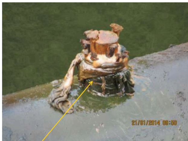
Close-up: Illegal fitting on 28" Nkpoku-Bomu Pipeline at Ekpoko. Picture was taken during Joint Investigation of 21st January 2014.
