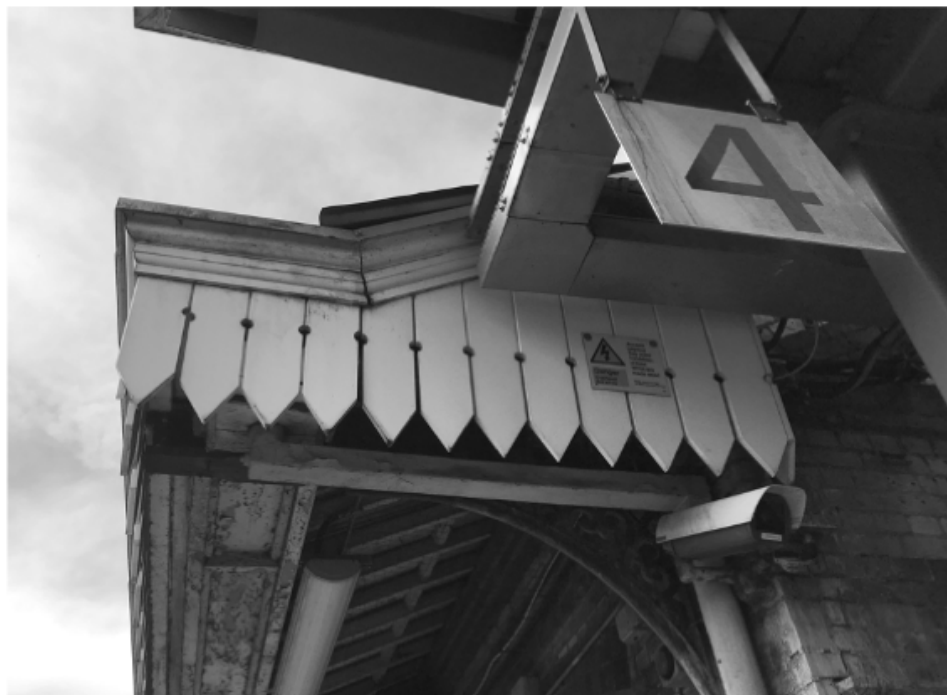
Figure 14 Canopy crenelations at Platform 4, Maidenhead Great Western Railway station UK. Note ‘drip-tips’ and circular reservoir between each pair of boardings hanging vertically down from roof. Twyford GWR station has pairs of daggerboard examples each with two vertically arranged ‘depots’.
