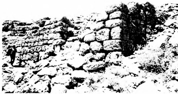
general view, looking southwest
