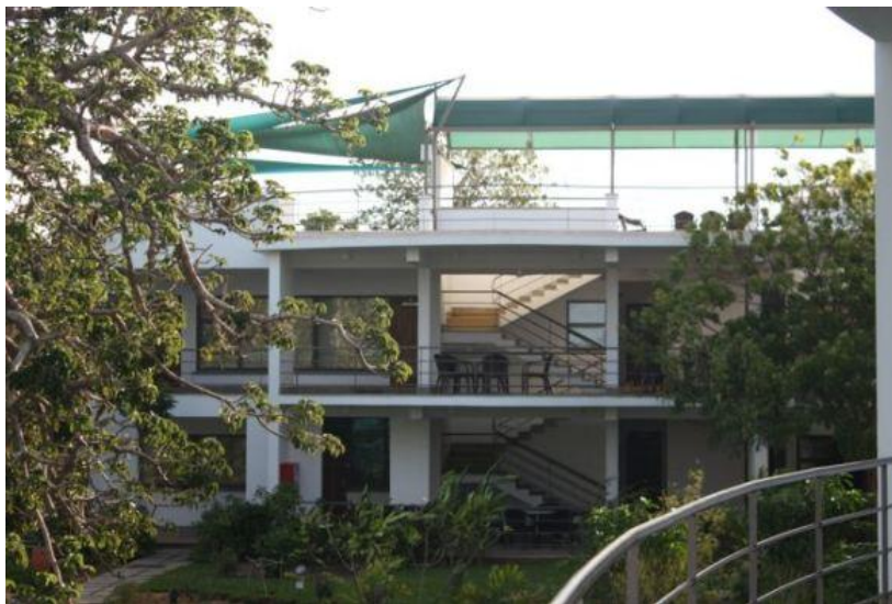
Figure 4: Picture of the main building of the KWTRP
