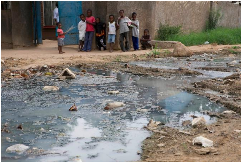
Figure 4. Raw sewage spills onto a street from a burst sewer main in the high-density suburb of Chitungwiza on the outskirts of Harare. Source: Jason Tanner Photography.
