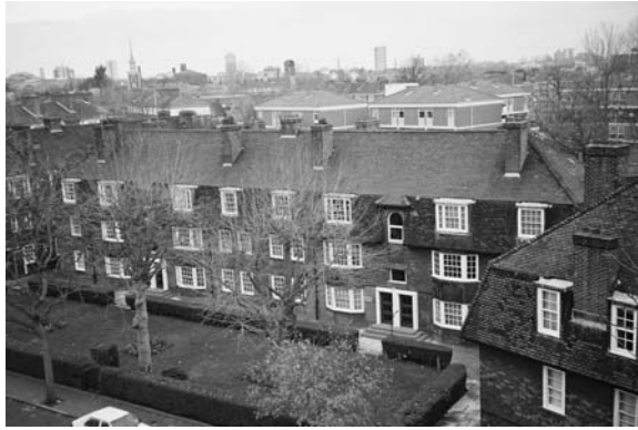
(a) Murdoch House from the South
