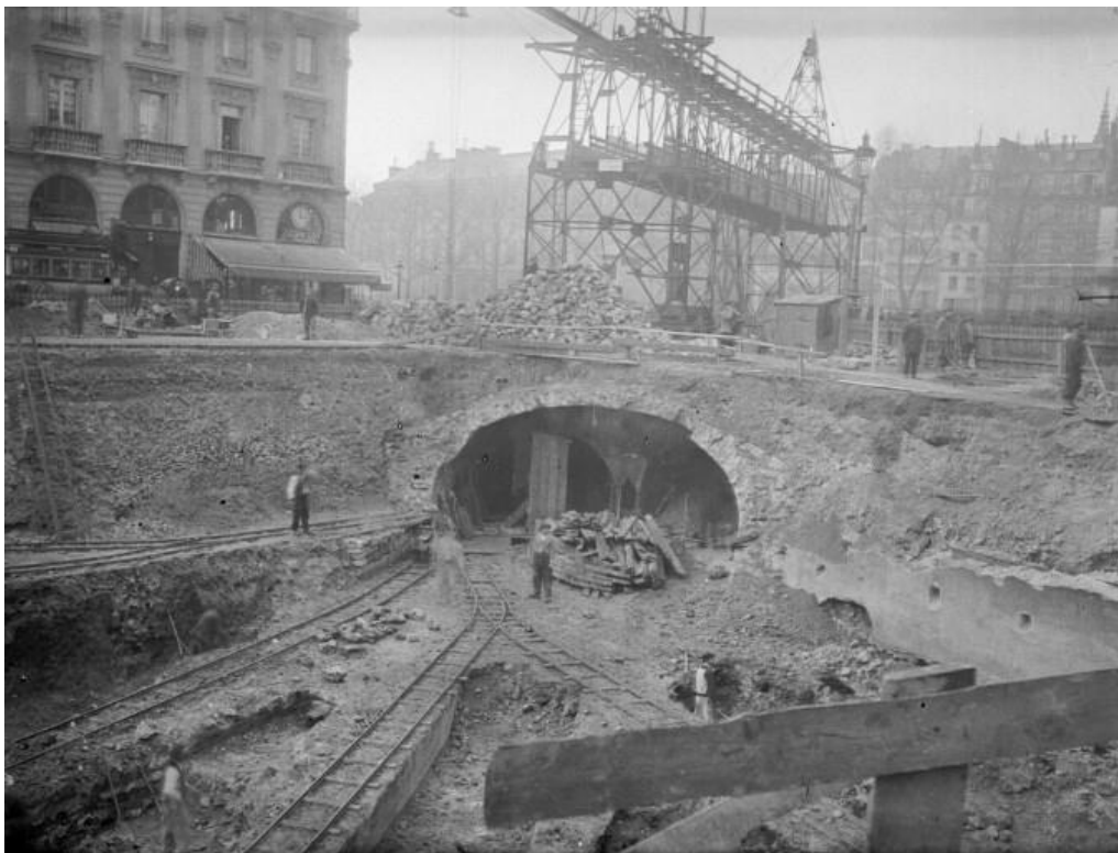
Illustration 7.2: The construction of the Métro 337
