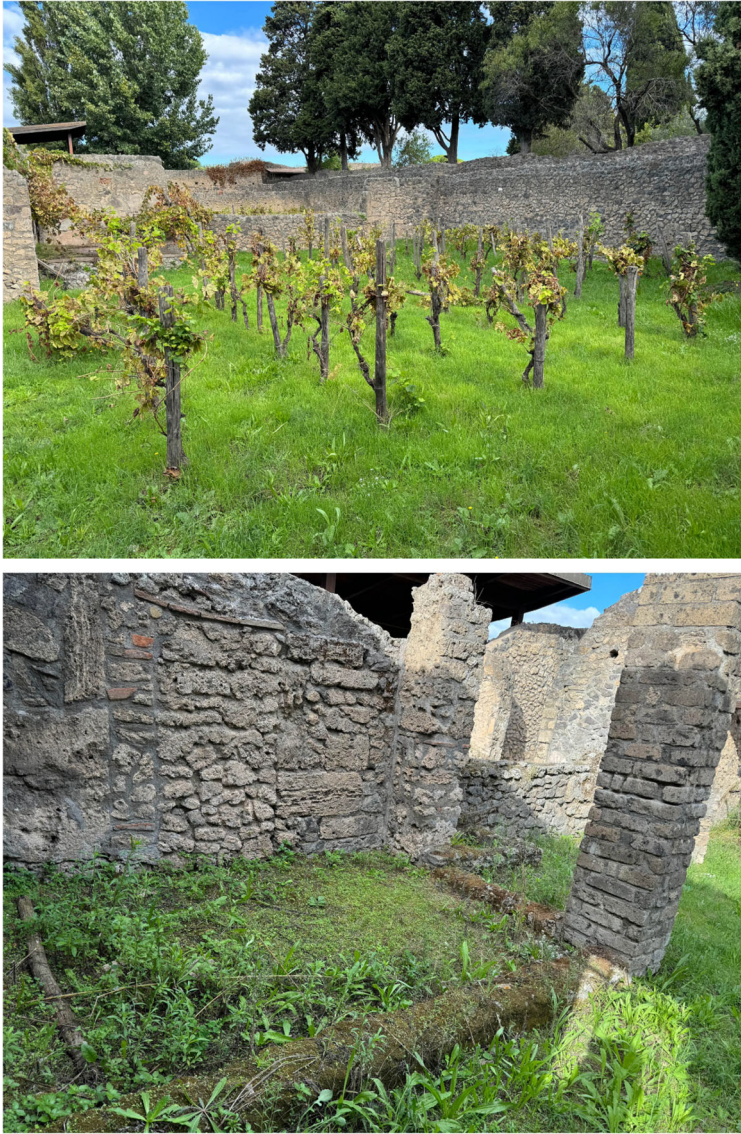
Fig. 8. The opportunistic garden at II.1.7B/8–9, viewed from entrance 8. The garden is now planted with a vineyard (top). A blocked door can be seen between the interior space and garden on the rear wall of the treading floor (bottom), to the left of entrance 8. (Image: Author's own/Archaeological Park of Pompeii.)
