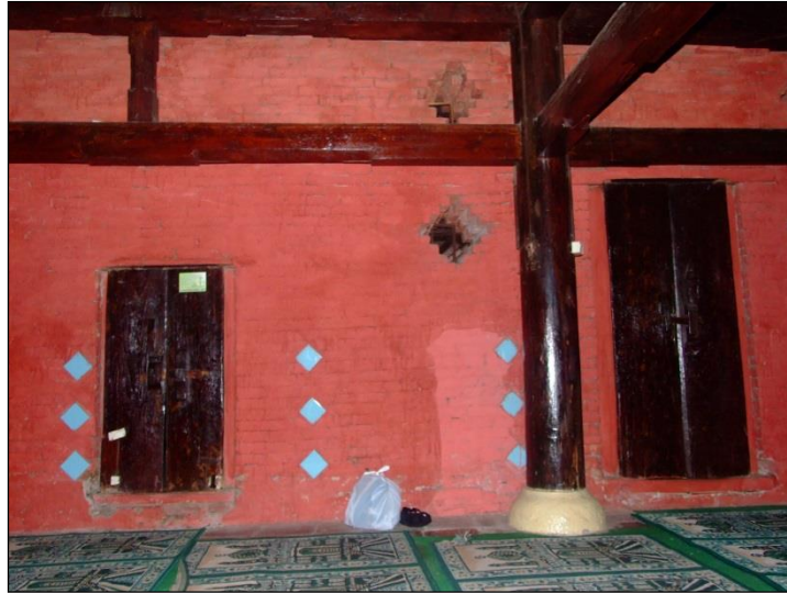
Figure 33: Two examples (large and small) of the Masjid Agung Cirebon's northern and southern doorways. Two diamond-shaped ventilation shafts are also shown. The blue tiles are modern.
