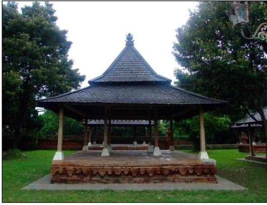
Figure 51: Example of a square pendopo , Keraton Kesepuhan.
