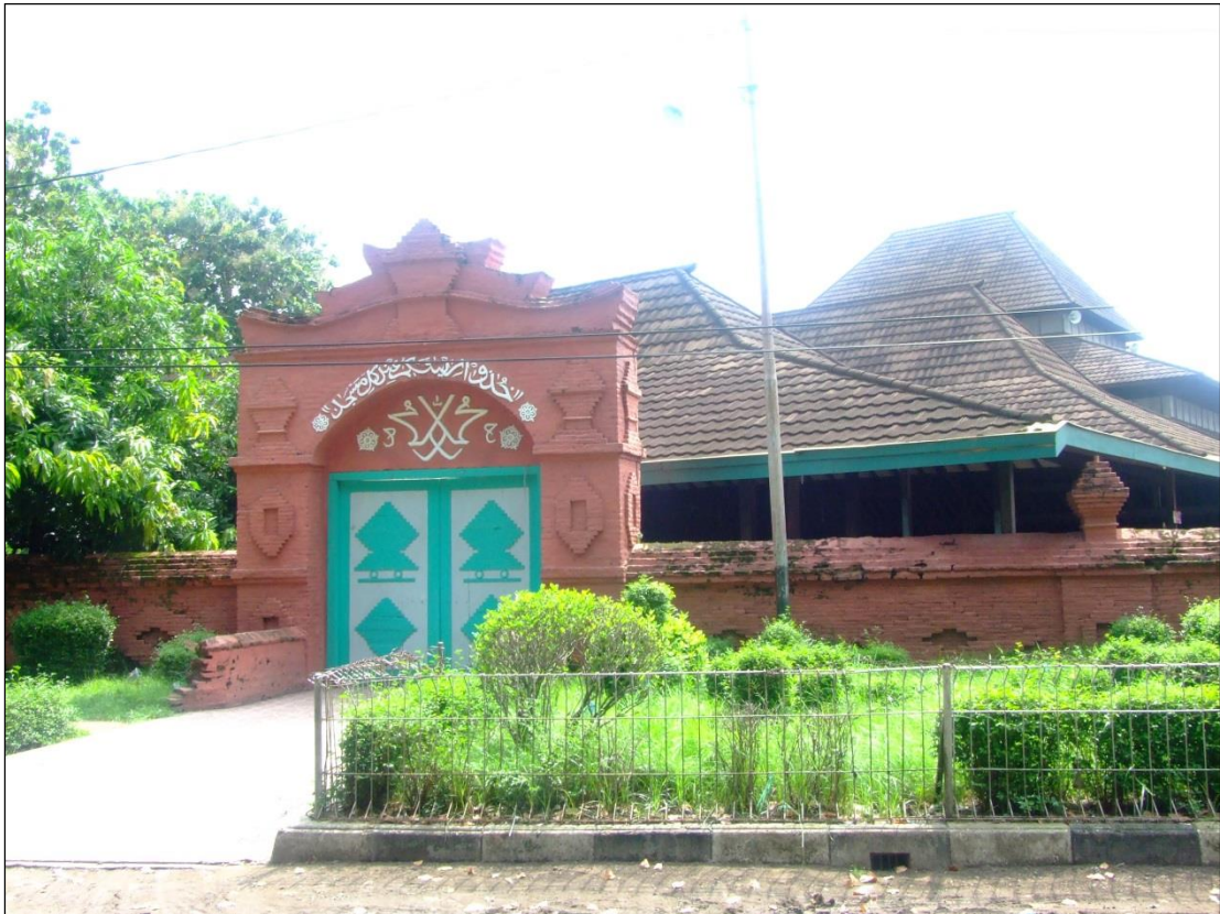
Figure 31: The Masjid Agung Cirebon complex. The mosque is the tall building located at the rear. The two buildings immediately behind the gateway are later serambi .
