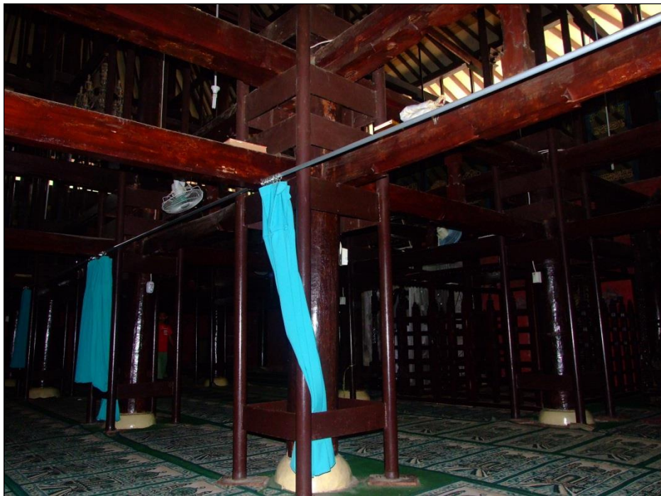
Figure 34: Interior of the Masjid Agung Cirebon's prayer hall, showing its columns, the lowest register of cross beams and the supporting steel structure.
