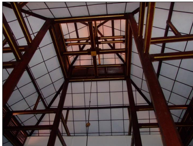
Figure 44: The Masjid Agung Banten's kingpost and cross beams.
