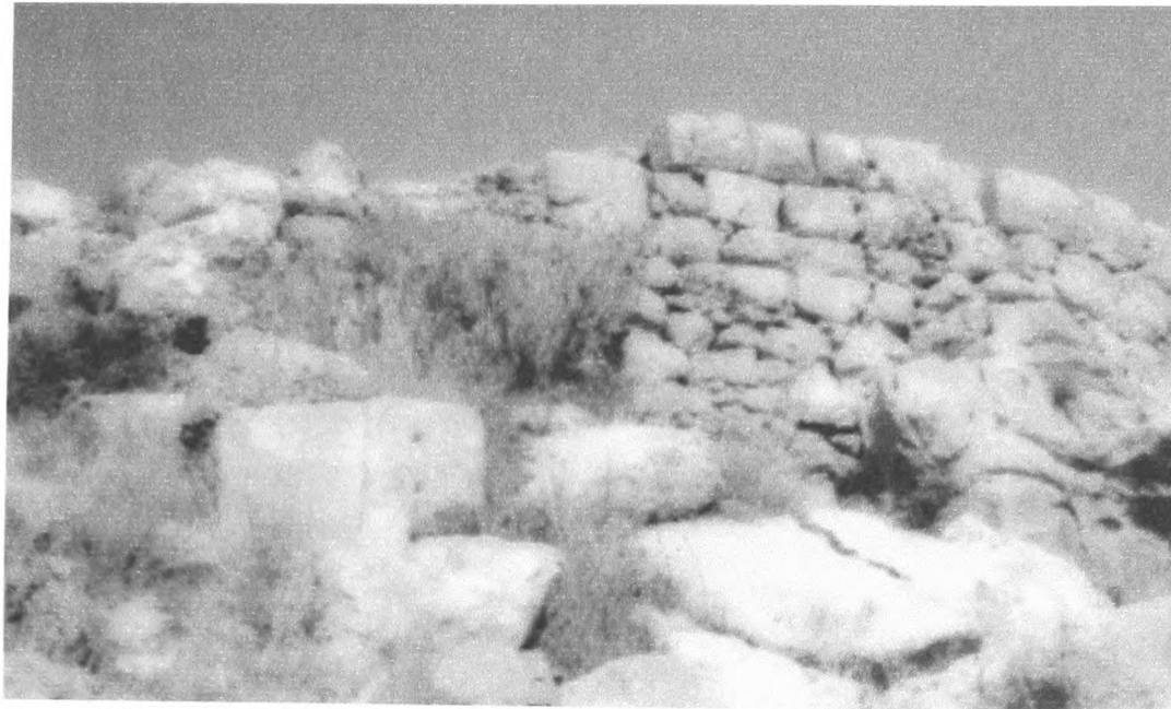
75. Ariassos, late fortification wall near house 23
