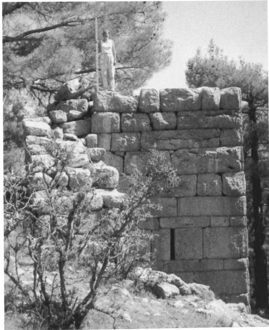
10. Sia, tower, T7, in fortification wall [B]
