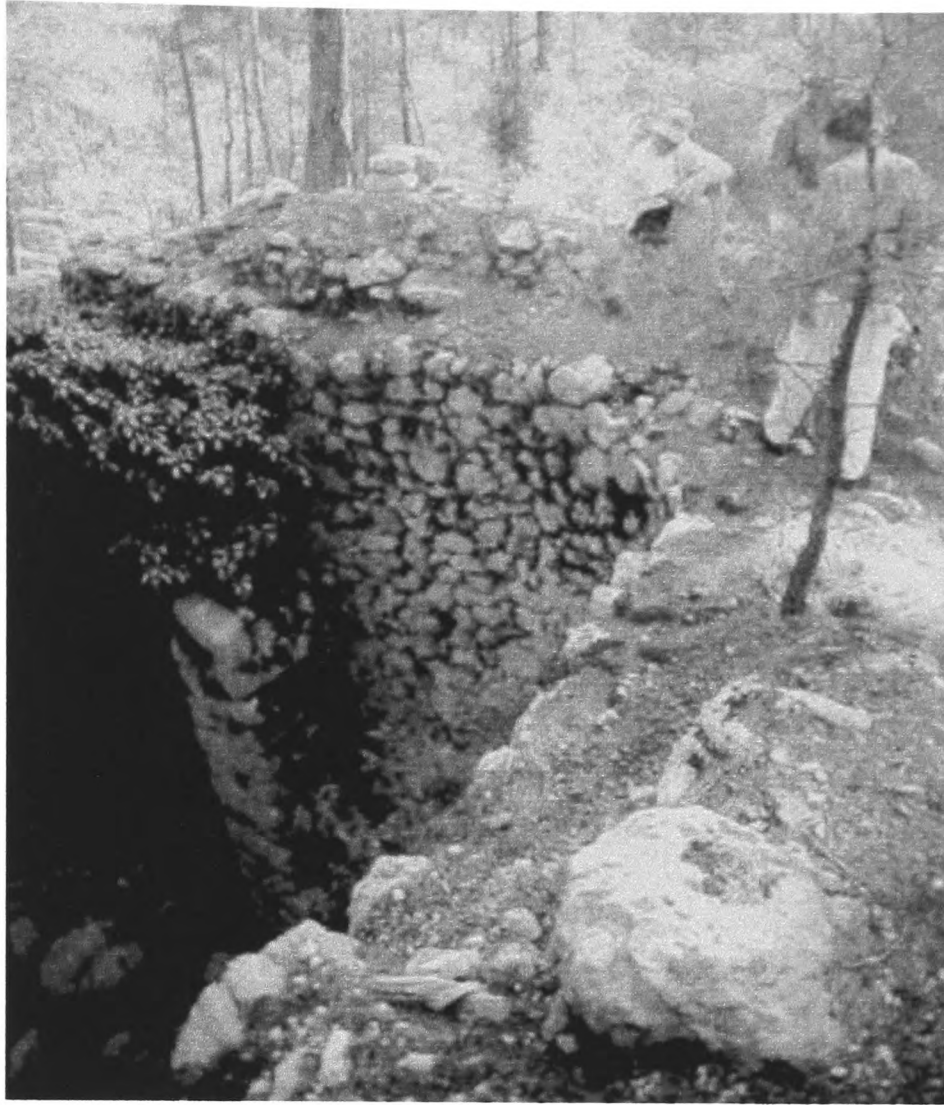
47. Sia, cistern above bathhouse
