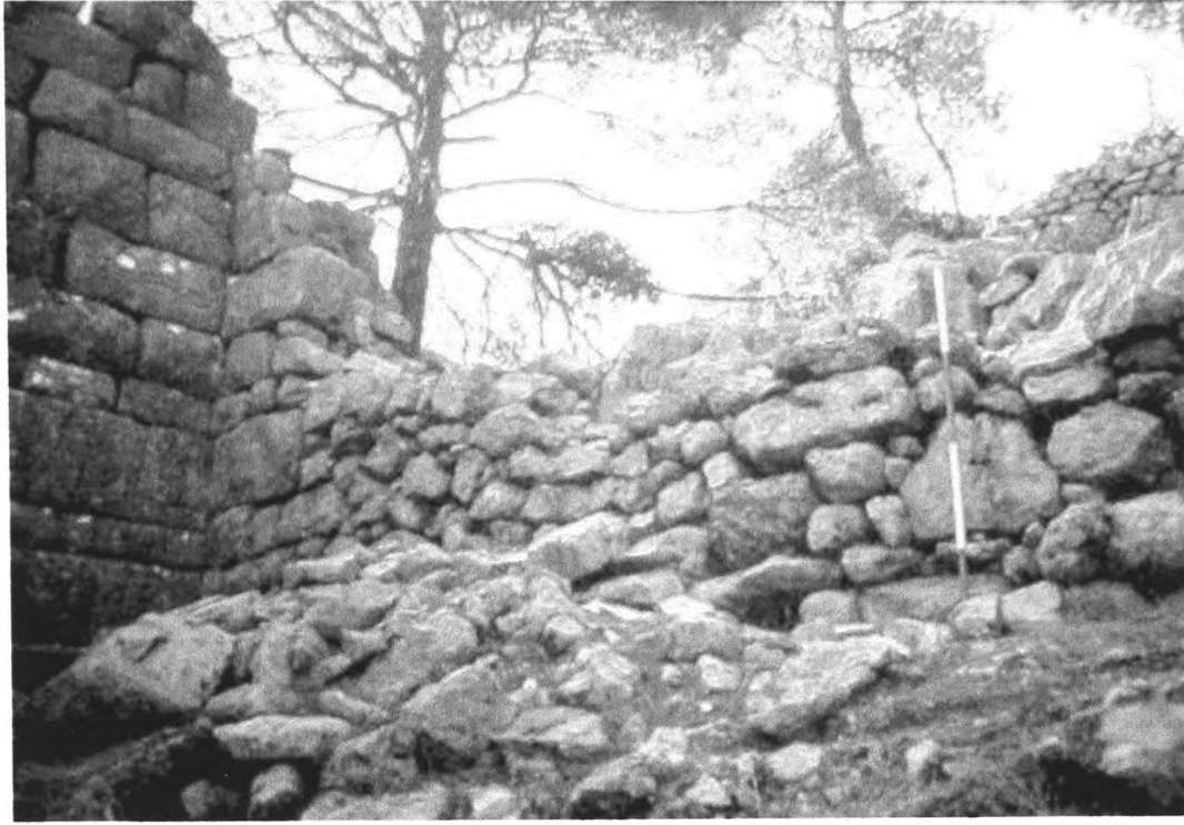
11. Sia, fortification wall [B] adjoining T7 showing repaired section
