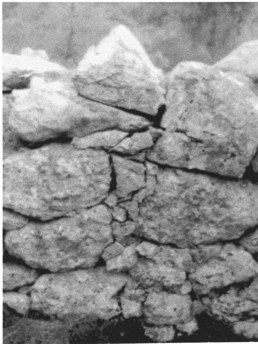
26. Ariassos, mortar in fortification wall north of house 23
