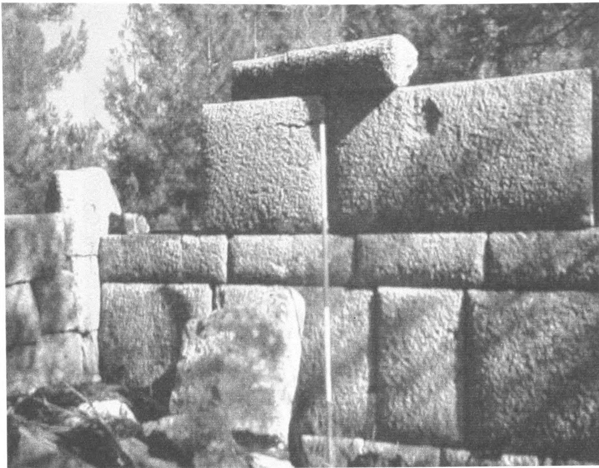
19. Sia, wall of Vm2 adjoining Vm3 (in left corner)
