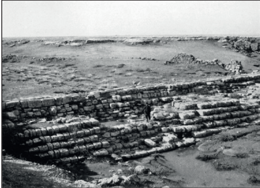
Fig. 5.13. Photograph of the stepped dam at Qasr Khabbaz (Gregory and Kennedy 1985, 195).
