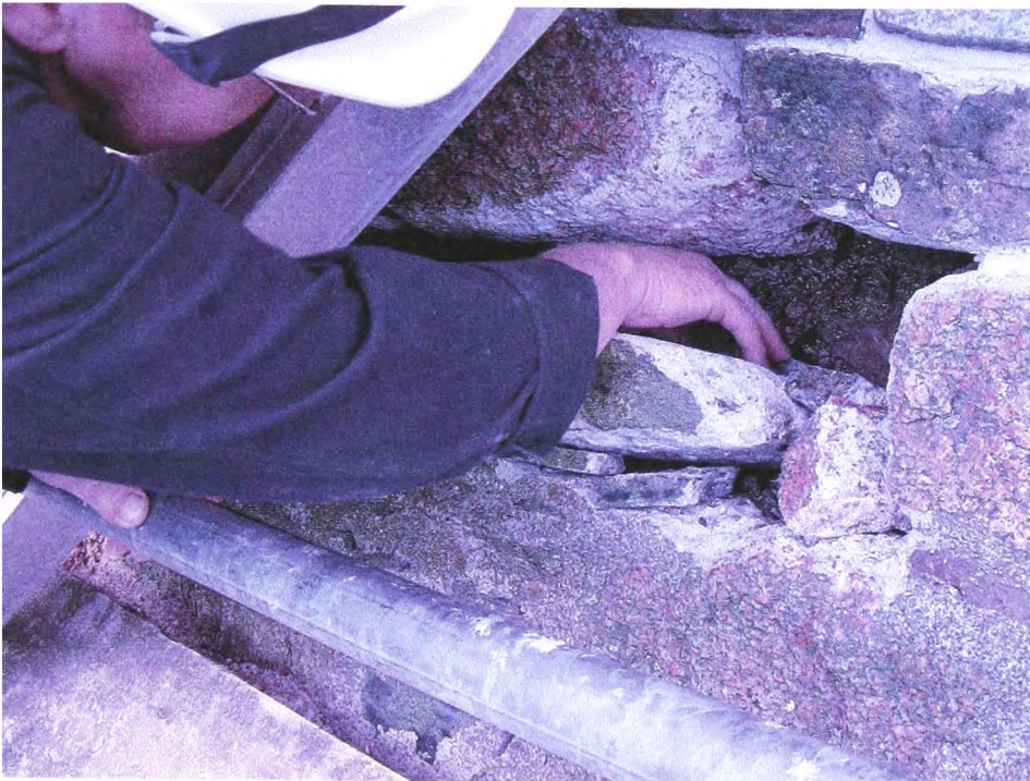
Fig 5.3 An MCU member repointing the Abbey church tower, exposing the original 12-century mixture of broken shells, lime, and ash
