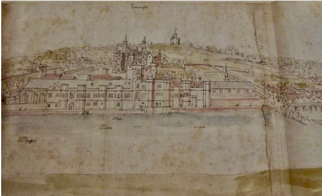
Figure 6. Detail from Anton van den Wyngaerde's 'Greenwich Palace', c. 1558 Ashmolean Museum, Oxford, WA. C. LG. IV. 8b. The image shows the steps leading to the river are shown to the left of the image, and the pier to the far right. Image: Author's own, by kind permission of the Ashmolean Museum.
