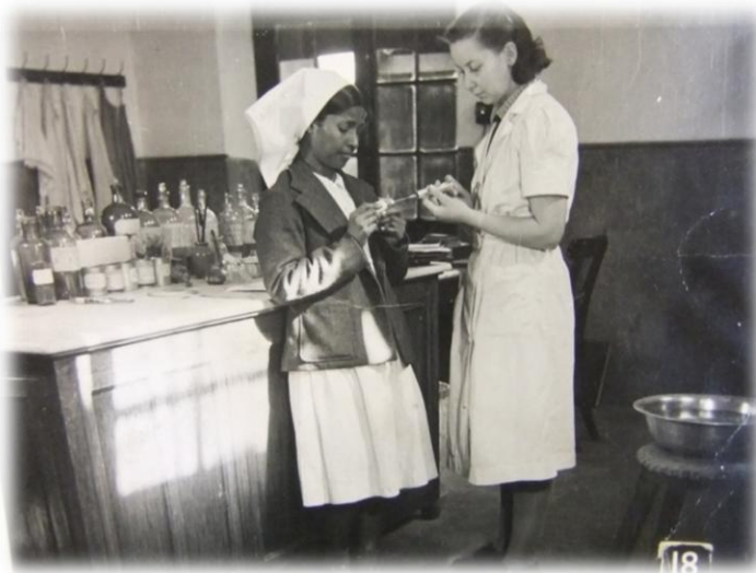
Preparing an injection
