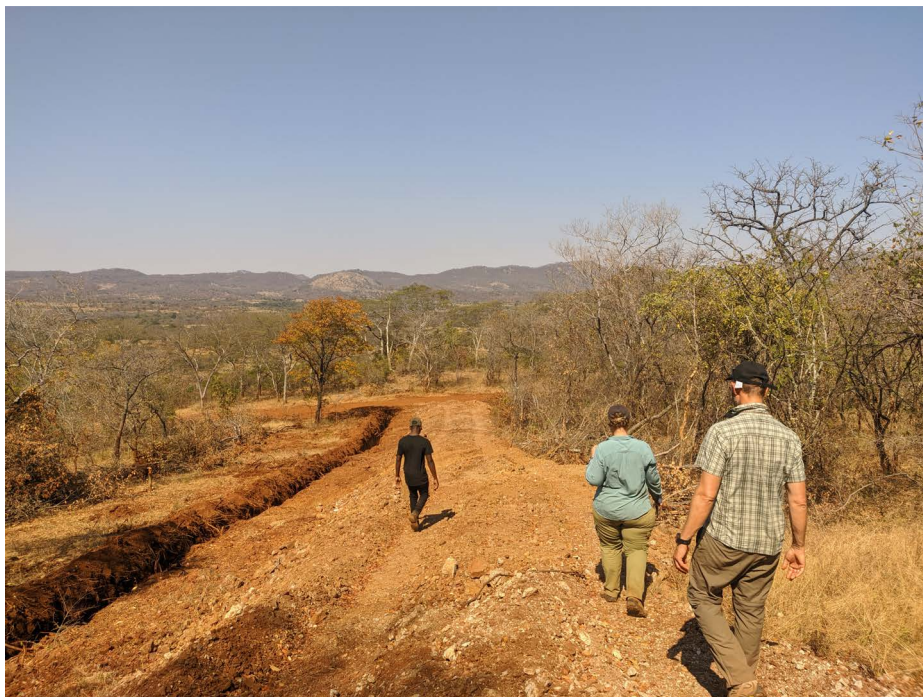
Figure B.12: Trench from which MO01-5 were collected, trenched by Li3 in the Odzi greenstone belt.
