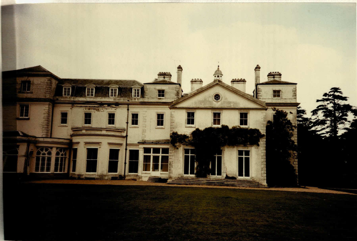
West and South Fronts
