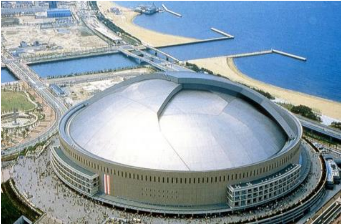
Figure 2.1.2: Fukuoka Dome with retractable titanium roof [1].
