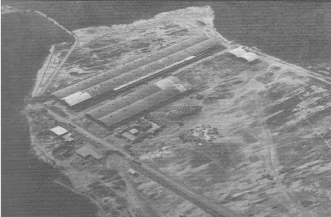
Figure 38: Photograph of Nichemtex Textile Factory, Lagos, built 1971-1973
