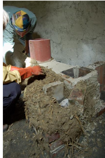
Home-made cement and mud rocket stove in production (source: bioenergylists.org )
