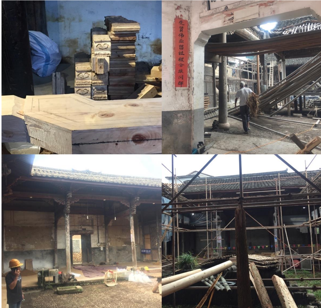
Figure 4: Renovation sites within the GMJ using 'traditional' materials Photo by Author
