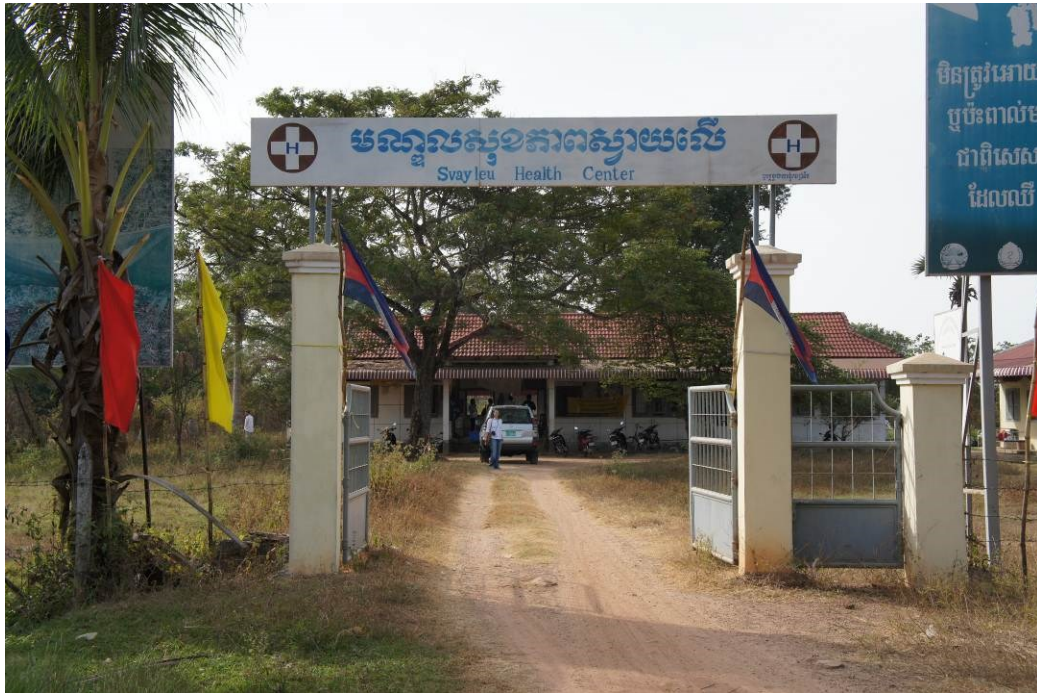
Figure 1.1-11. Government Health Centre in Siem Reap Province, Cambodia.
