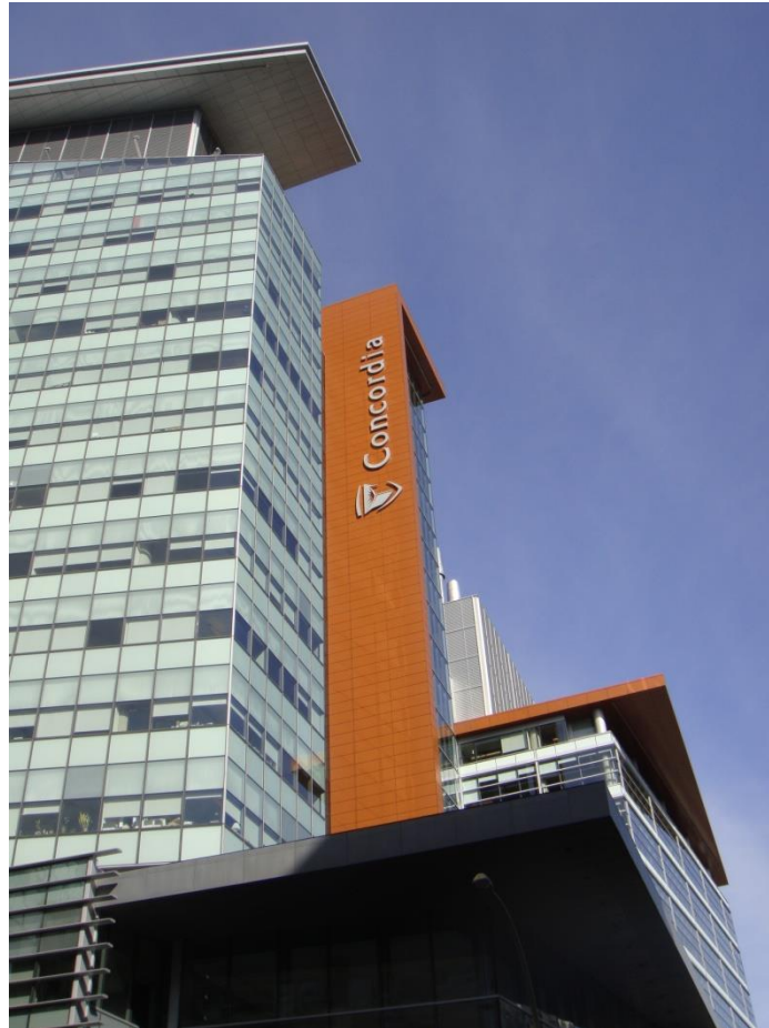
Figure 2: The 'EV' Building, Concordia University
