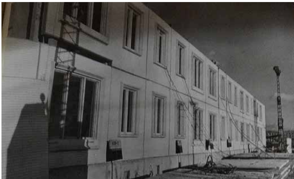
Fig. 1.7 a-c Methods of construction used in the 9th district of Cheremushki: a. brick construction (buildings 1–13 Б, В); b. large-block method (building 13); c. large-panel method (building 14). Source: RGAS, f. P-149, o. 1-1, d. 241, ll. 15, 26, 27.
