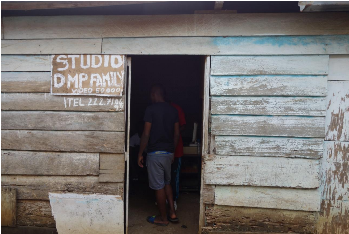
Figure 8.6: Exterior of DMP Family studio. (Source: author)
