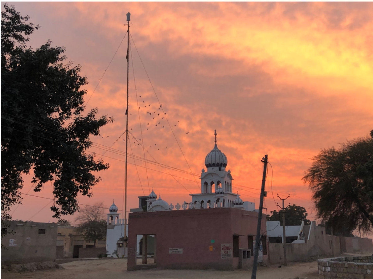
Figure 1.3. A Sikh gurdwara and Nishan Sahib (saffron Sikh flag and flagstaff) in a village in Padampur tehsil.
