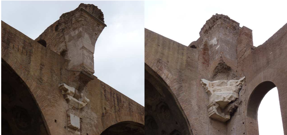
Fig. 2.13. Remains of the north side springings of the lost cross vaults over the central space of the Basilica of Maxentius: axis B (left) and axis D (right).
