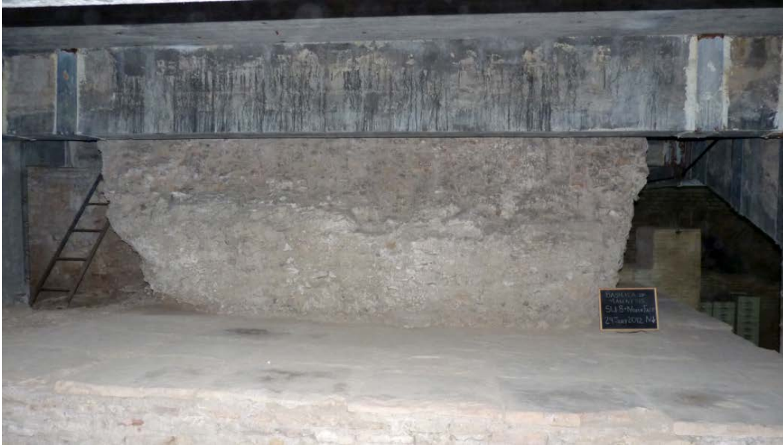
Fig. 3.11. Photograph of the Roman concrete foundation for the decorative column in front of the pier.
