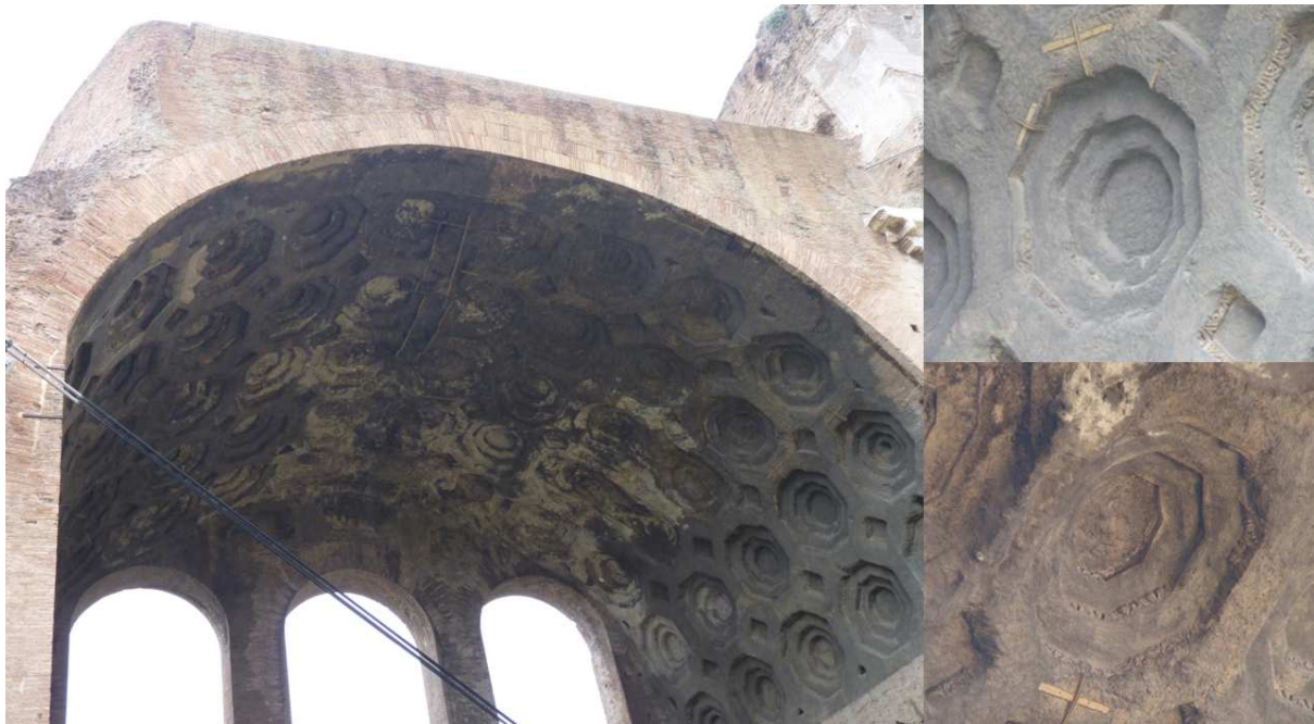
Fig. 2.4. Coffering decoration on the intrados of the barrel vaults of the Basilica of Maxentius. Left: west vault; right, up: detail of repaired coffering; right, down: detail of wear in ribs around coffering.
