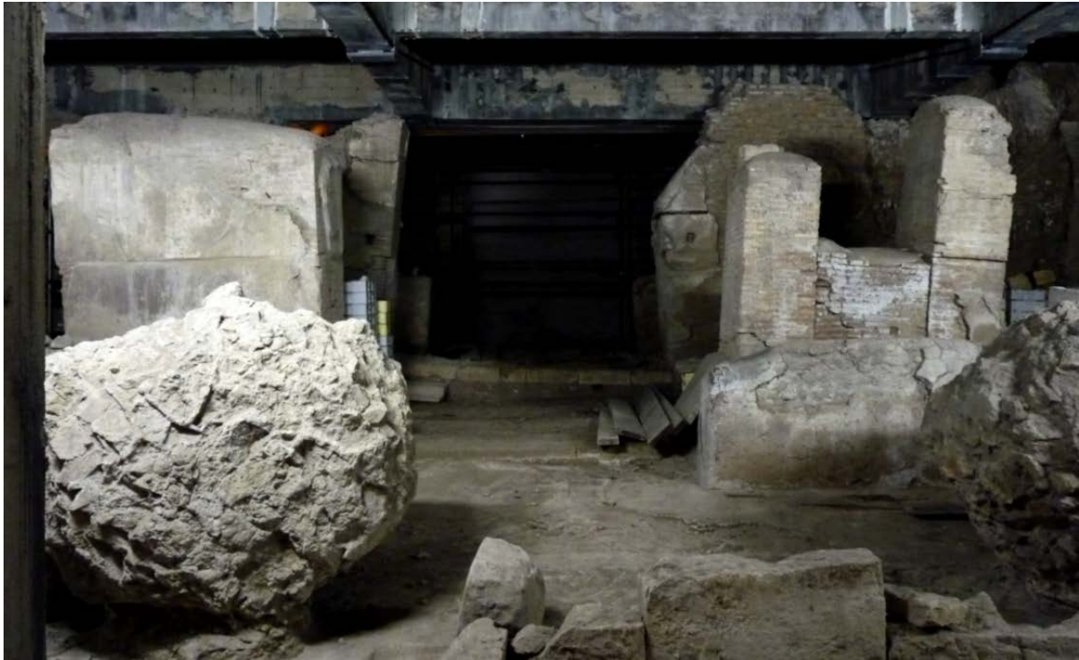
Fig. 3.8. Remains of four piers of the Horrea Pipperataria inclined in opposite directions. A sign that they have been exposed to lateral loading, probably oscillating seismic loading (photo: Albuerne 2012).
