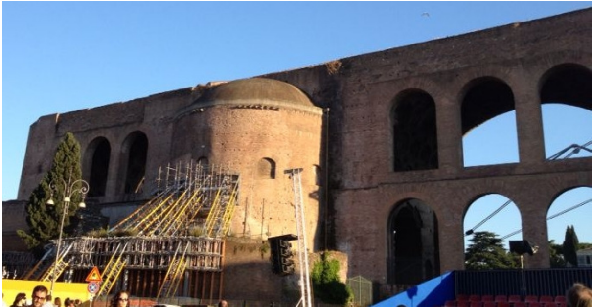
Fig. 1.6. Temporary propping of the north apse of the Basilica of Maxentius during the construction of a metro station and line a short distance from the monument (photo: Macaro, May 2014).
