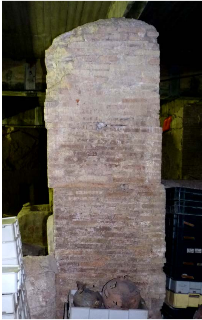
Fig. 3.9. Surviving wall of the Horrea Pipperataria showing slip at un-bonded bipedale layers, sign of horizontal loading (photo: Albuerne 2012). This type of damage is often observed in monumental ashlar columns, today free-standing, that have suffered damage in an earthquake.
