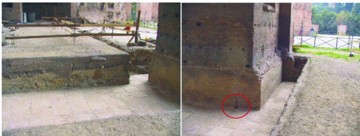
Fig. 3.1. Photographs of excavations of the foundations of the piers on the north nave of the Basilica of Maxentius in the late 1990's. Top layer of foundation structure exposed: levelled horizontal plane with bipedale finishing (photos: Cardarelli 2009).
