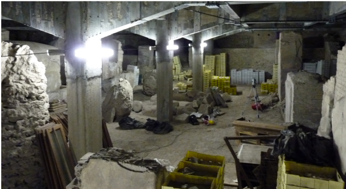
Fig. 3.5. Excavated basement space under the south nave of the Basilica of Maxentius, looking west (above) and looking east (below) (photo: Albuerne 2012).
