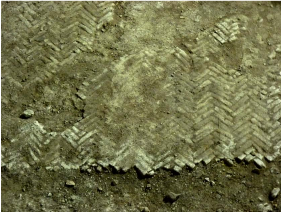
Fig. 3.6. Opus spicatum on the floor of Horrea Pipperataria (photo: Albuerne 2012).
