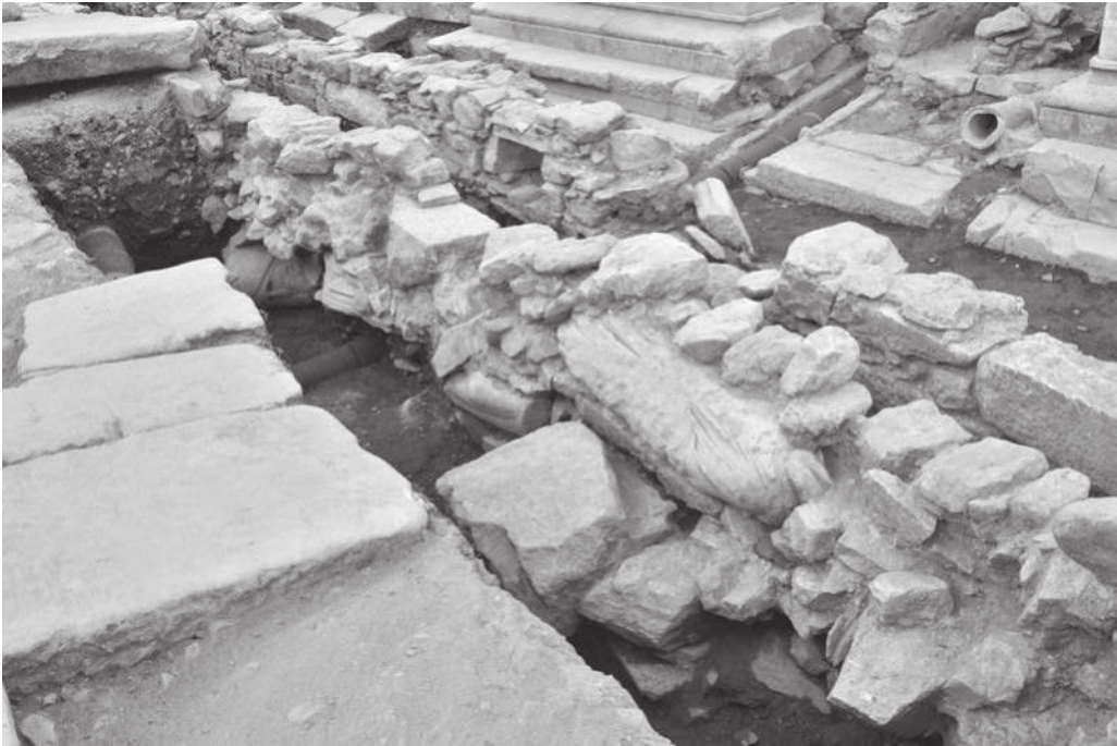
Fig. 12.2: Sixth-century street drain constructed with mortared rubble and statuary fragments (© Aphrodisias Excavations).
