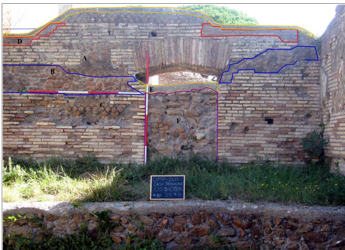
Figure 6.11. Opus reticulata wall in Casa Basilicale, showing multiple reconstruction phases and repairs. A – original phase reticulata, intact; B – degraded reticulata has been replaced with rubble; C – original phase reticulata, degraded; D – later-phase brick work repair; E – consolidation; F – rubble in-fill of blocked doorway. Scale rods = 2 m. Photograph by author.
