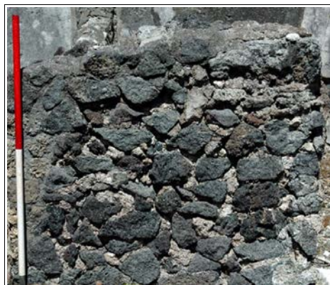
Figure 2.3: Unfaced rubble work in Casa delle Vestali, Pompeii, similar to the opus incertum facing style found in Ostia. B. Photograph by author.
