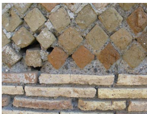
Figure 5.1: Example of reticulate facing, showing intact mortar at the interface between reticulate blocks and course of bricks. Lighter grey re-pointing mortar is visible at top of photo. Photograph by author.
