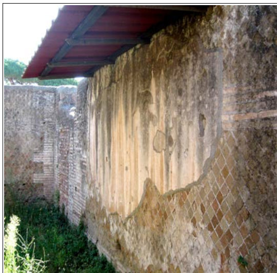
Figure 6.3. The remains of decoration covering wall with brick and reticulate facing in Case a Giardino, showing the carefully crafted pattern of reticulate and brick courses, both covered with plaster. Photograph by author.
