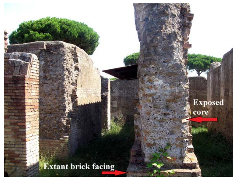
Figure 2.1: Remains of concrete walls in Casa a Giardino, Ostia, showing and fragments of extant brick facing on lower third of wall and the exposed wall core with coarse rubble aggregate. Photograph by author.
