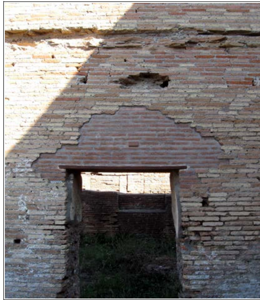
Figure 6.5. Repair over a doorway in Caseggiato del Serapide, showing new bricks set back from the original construction area. Photograph by author.
