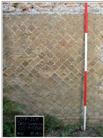
Figure 2.4: Reticulate pattern of tuff blocks, Casa a Giardino, Ostia. Photograph by author.
