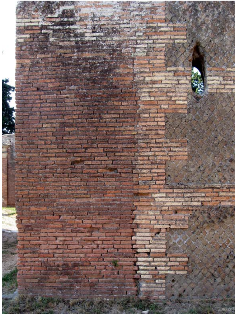
Figure 6.27. Discontinuity in brick types, Piccolo Mercato. Photograph by author.
