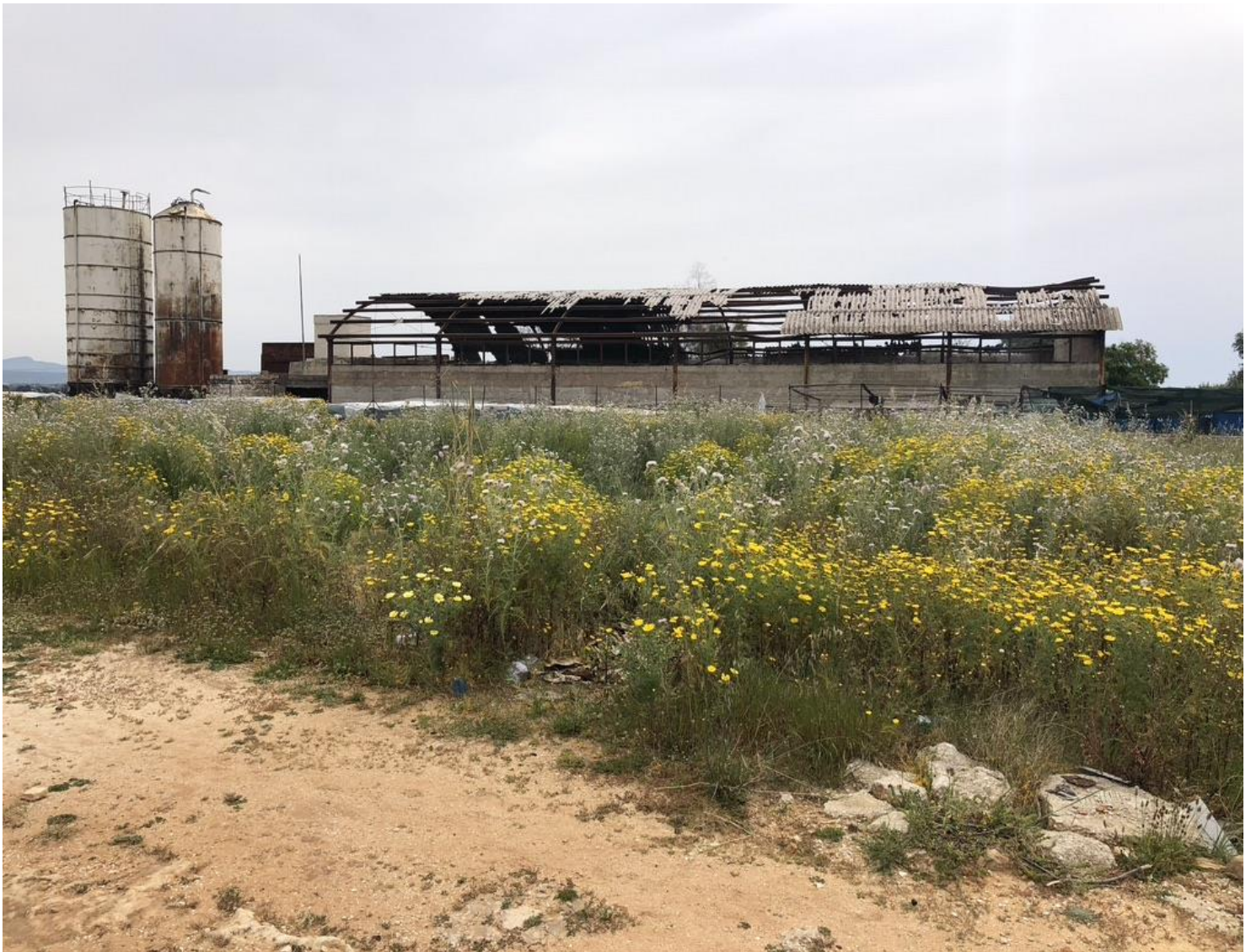
Figure 22 The former cement factory, seen from afar (photo by author)
