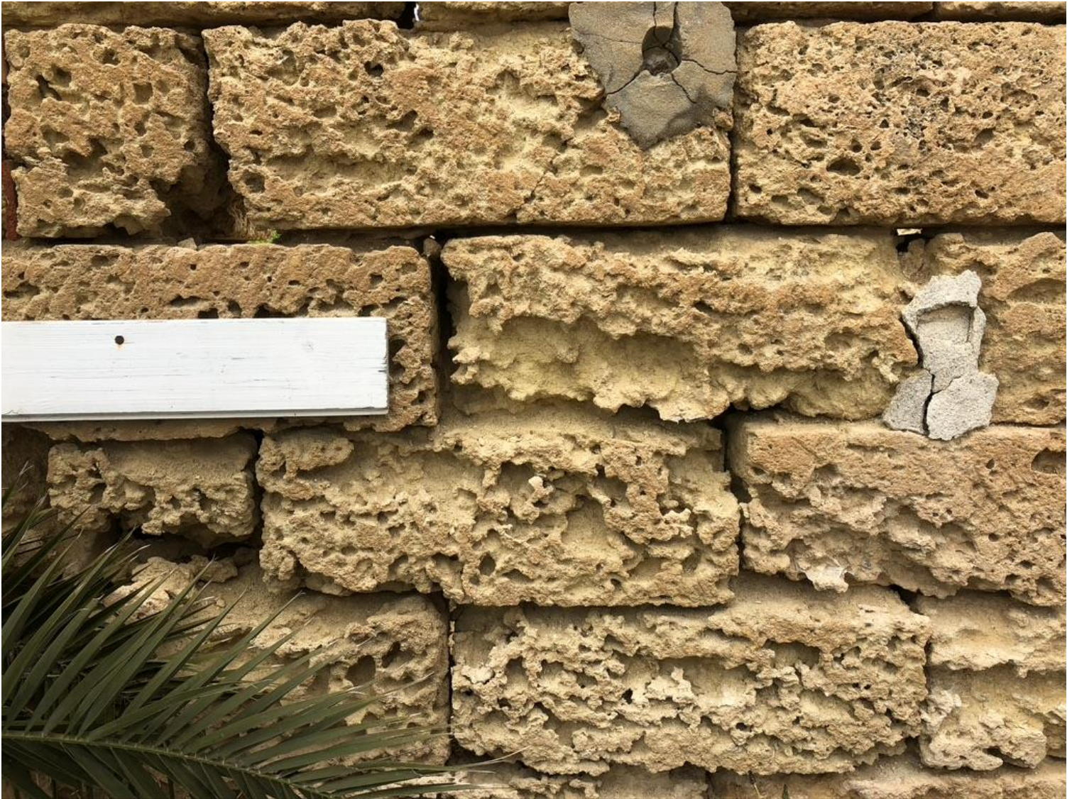
Figure 10 Tuff building, up close (photo by author)
