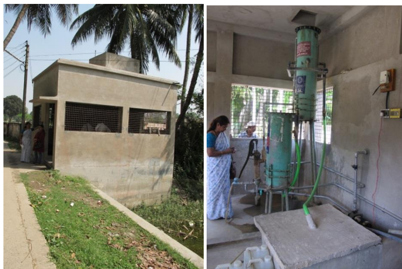
Photos: BESU 3:3 from the outside and inside.
