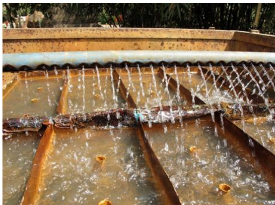
Photo 1.3 Aeration of raw water before the adsorption occurs on the iron nails
