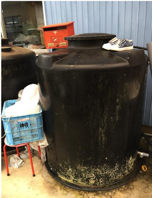
Photo 3: Water tank next to the shack of TITP labourers in Tokushima Prefecture
