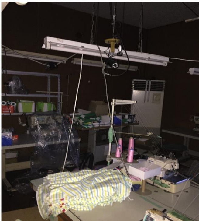
Photo 2: Surveillance camera at the garment factory (provided by Tokushima Roren)
