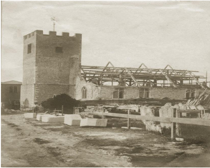
Figure 31 - Exterior during restoration.
