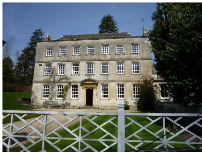
Fig 3.7: Pitchcombe House, c. 1743.
