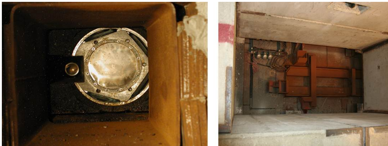
Figure 7.24: (left) Photo of the front face of the beam dump as taken in 2003. (right) Looking down on the top of the dump plug below the surface of the shielding blocks .
