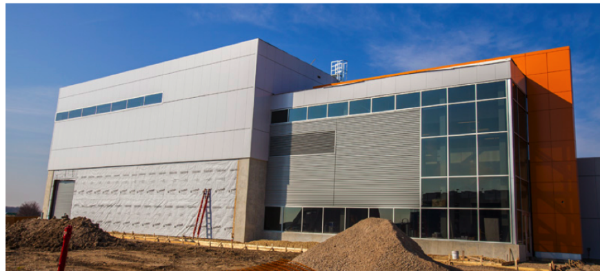
Figure 1.5: The completed MC-1 building in May 2014.
